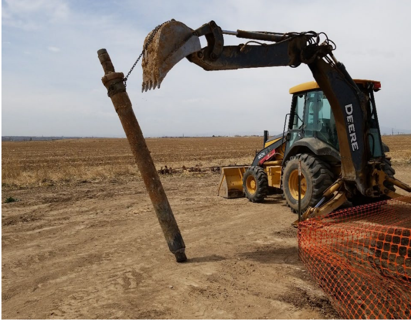
Lifting the cut casing.
