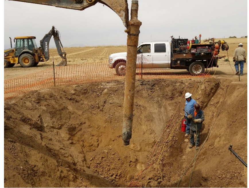
Lifting the cut casing.
