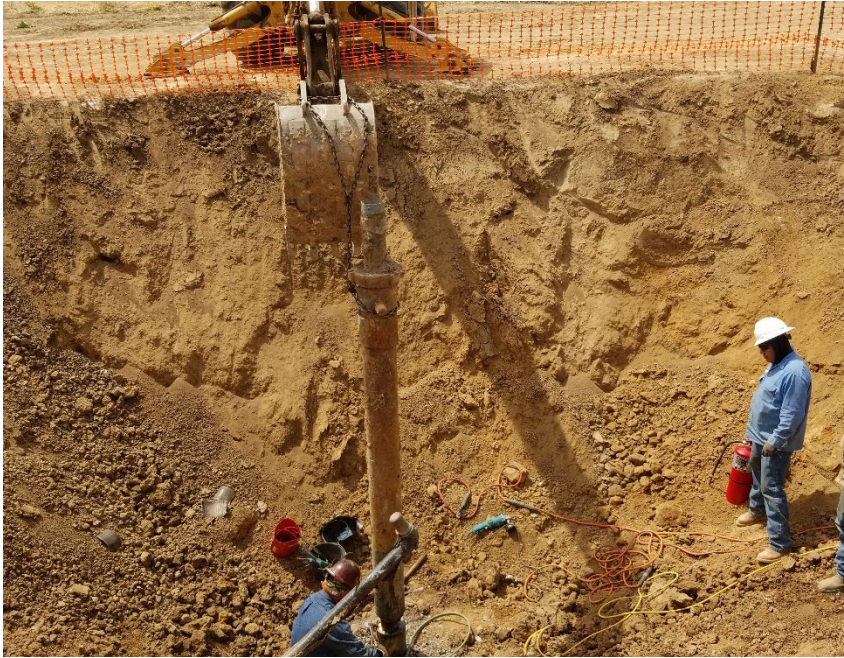
Lifting the cut casing.
