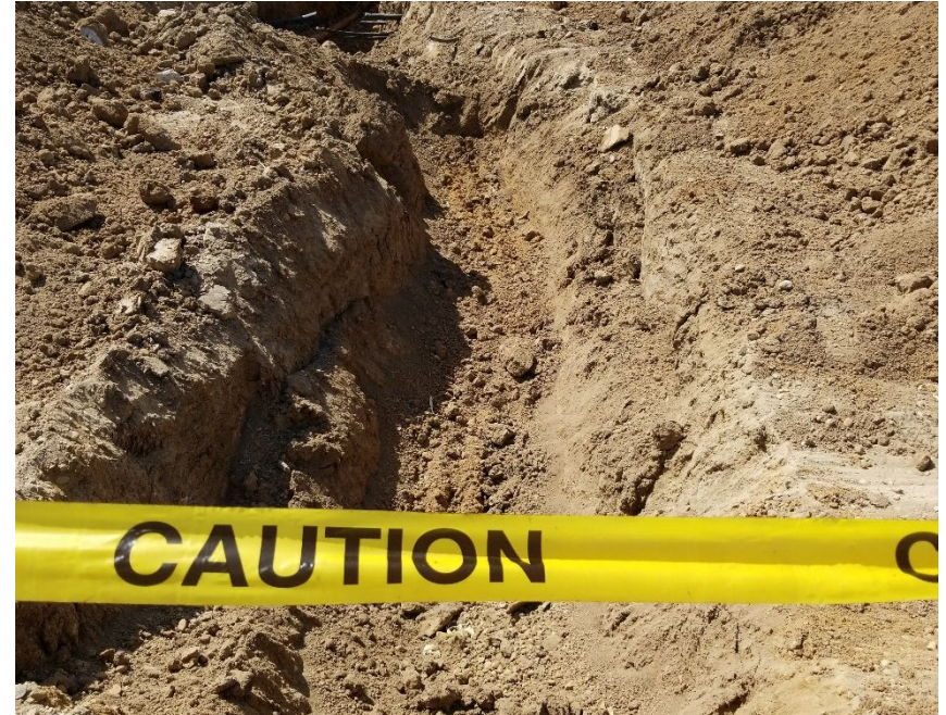
Open excavations with inadequate fencing.
