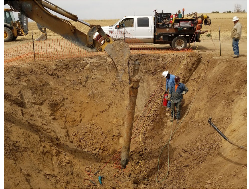
Lifting the cut casing.
