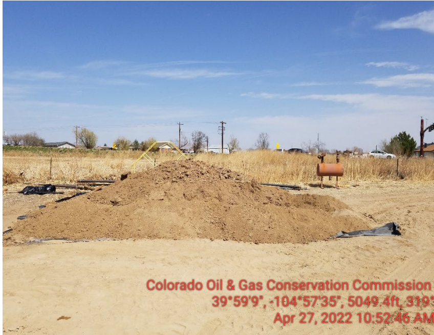
One of several spoils piles with inadequate stormwater BMPs.
