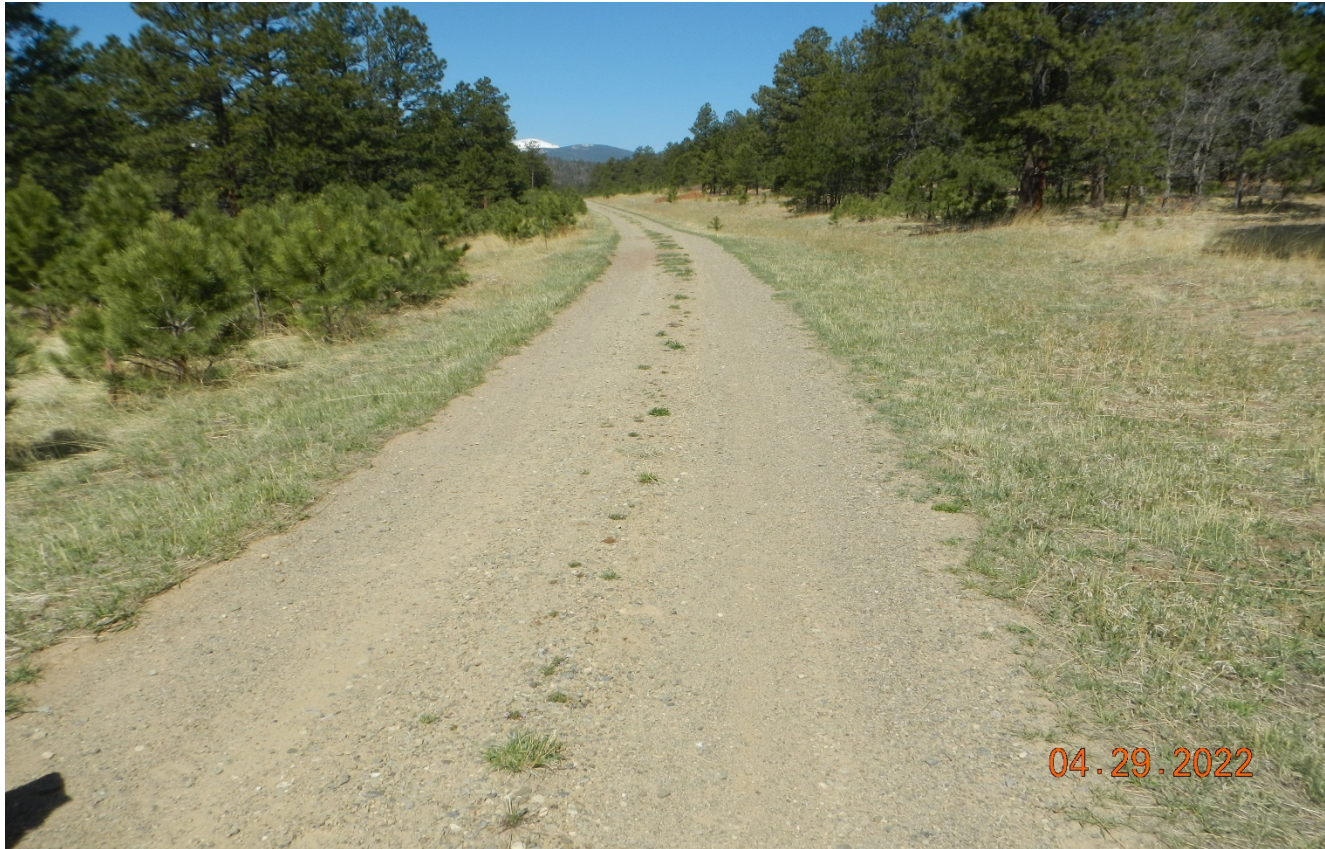
Photo 1. Facing west along the access road. The road is stabilized with gravel and vegetation.
