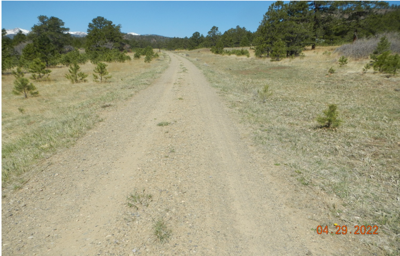
Photo 3. Facing west along the access road. The road is stabilized with gravel and vegetation.
