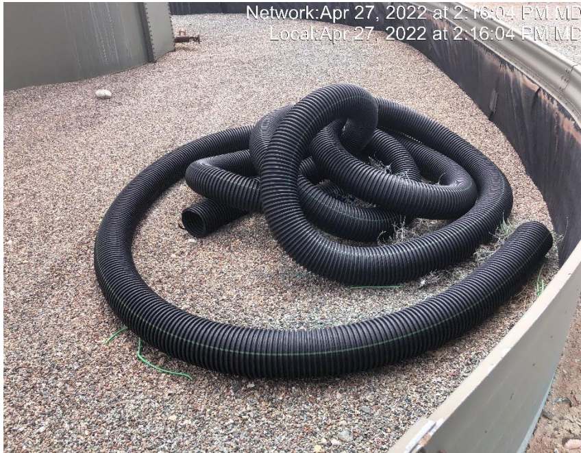
Photo #6571 Unused equipment in tank containment.
