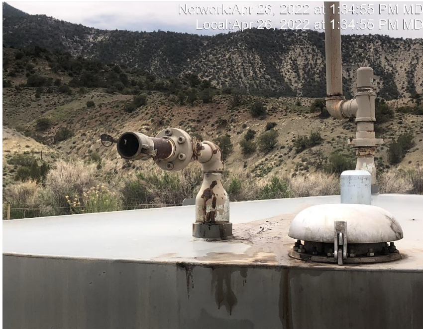
Photo #6558 Vent pipe on tank open ended.
