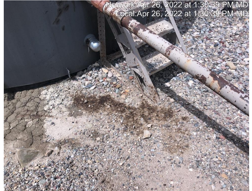
Photo #6557 Stained soils inside tank containment.
