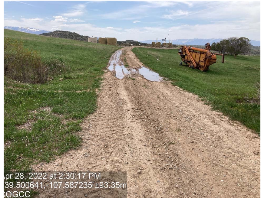
Lack of stabilization/compaction and irrigation run on
