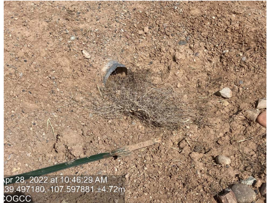
Culvert failing
