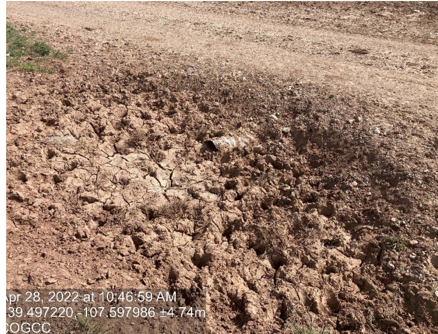
Culvert failing
