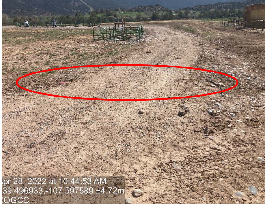
Culvert failing
