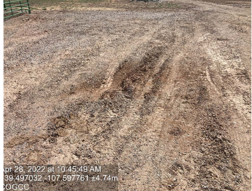
Lack of stabilization/compaction
