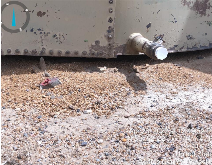
Photo#9 Gap under production tanks
