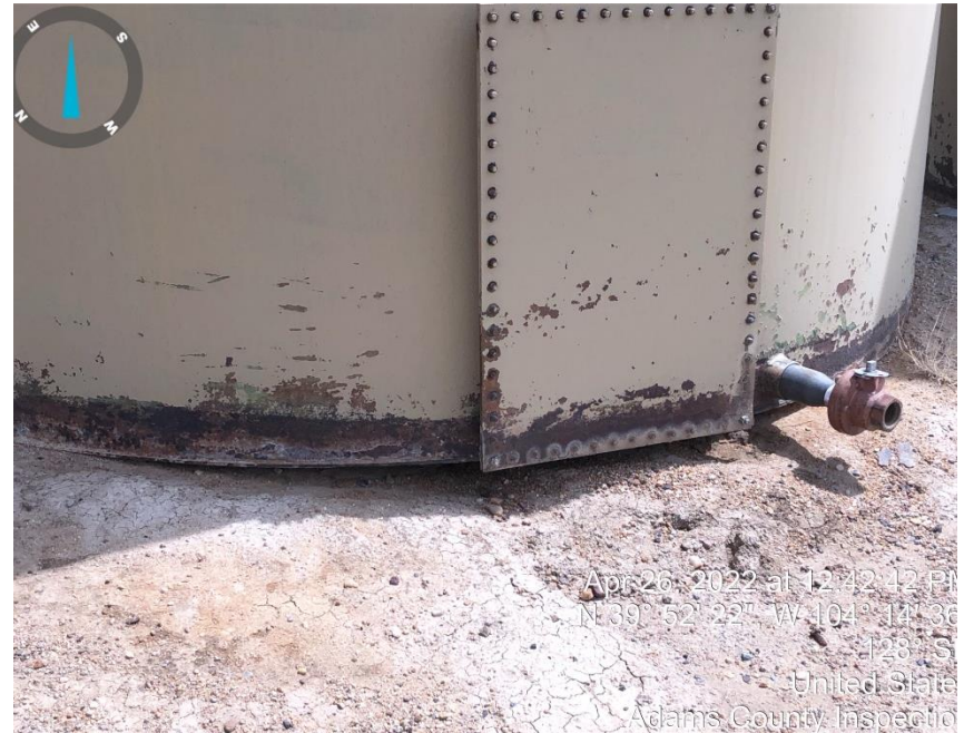
Photo#8 Gap under production tanks
