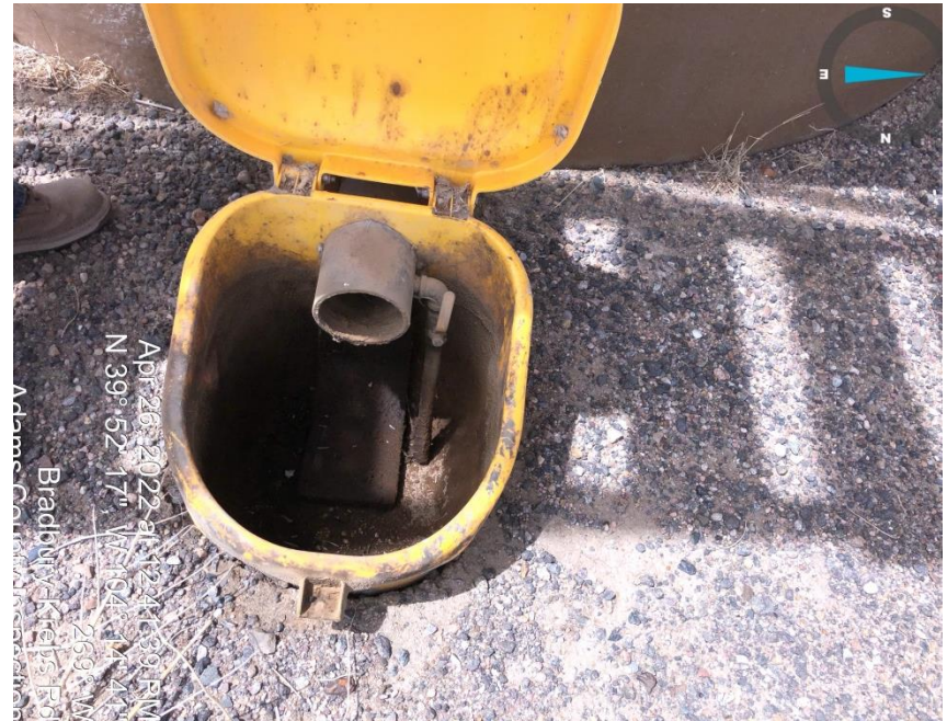
Photo#4 No bull plug on load out line.
