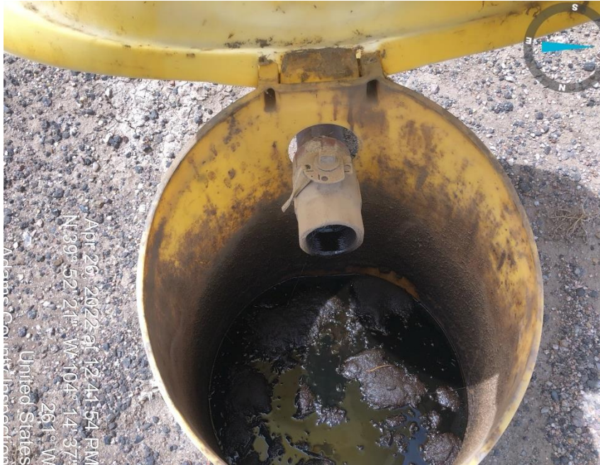
Photo#5 No bull plug on load out line.
