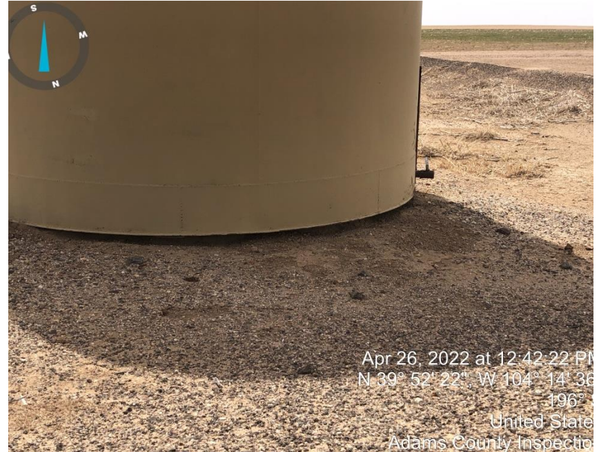
Photo#6 Gap under production tanks
