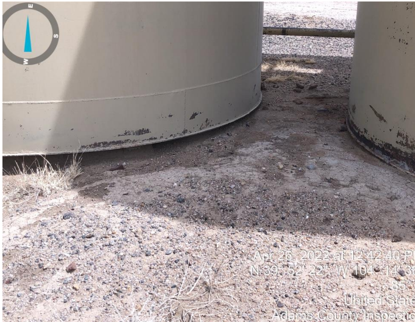
Photo#7 Gap under production tanks
