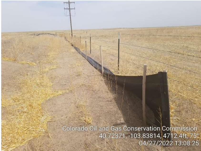
Photo 19 – Silt Fence in disrepair
