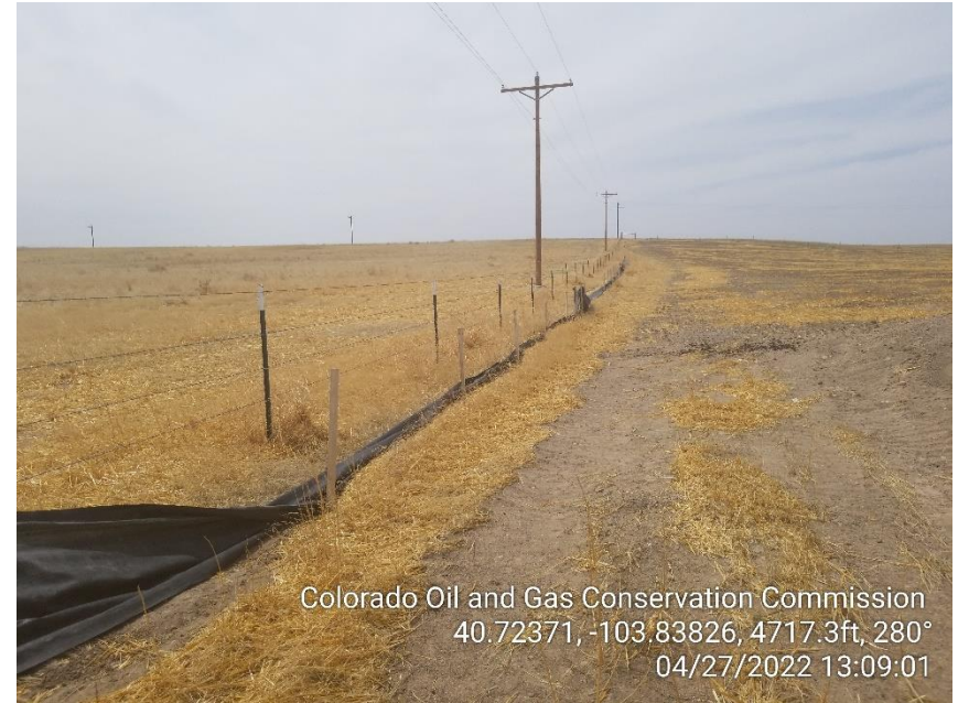
Photo 20 – Silt Fence in disrepair
