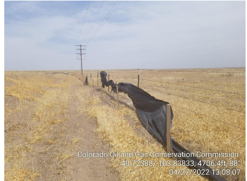
Photo 18 – Silt Fence in disrepair
