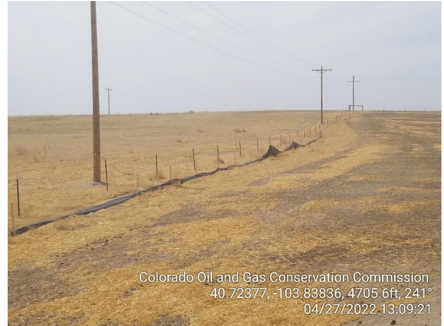
Photo 22 – Silt Fence in disrepair
