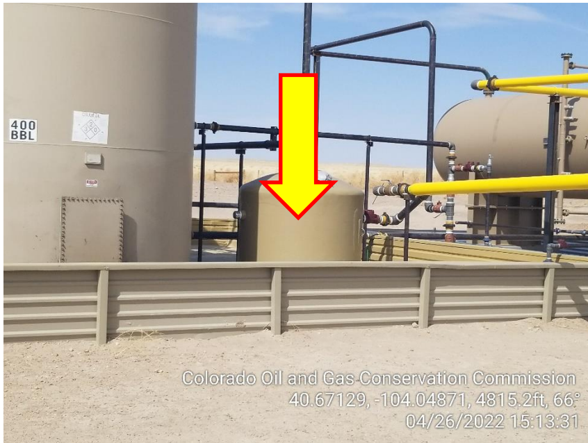
Photo 5 – Tank missing Labels
