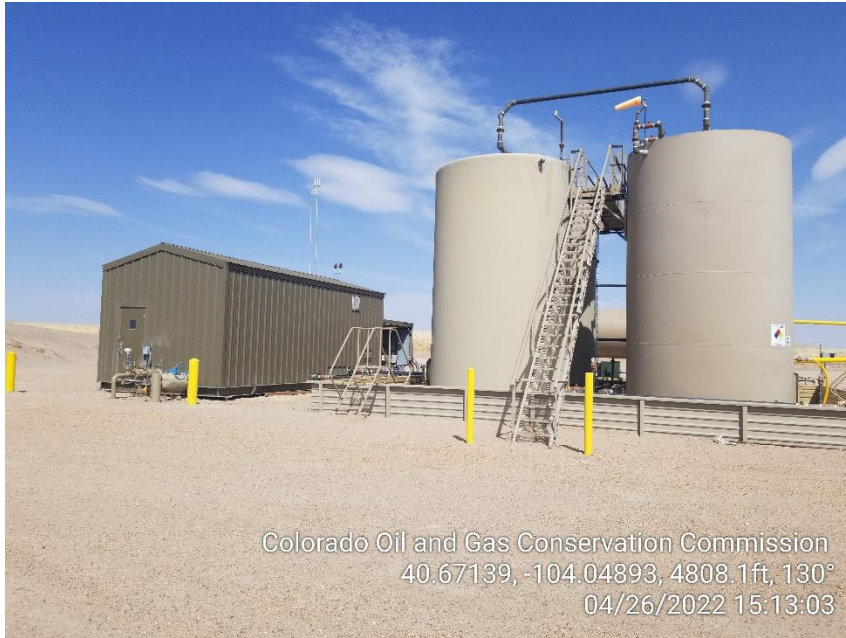
Photo 3 – Tank Battery and LACT
