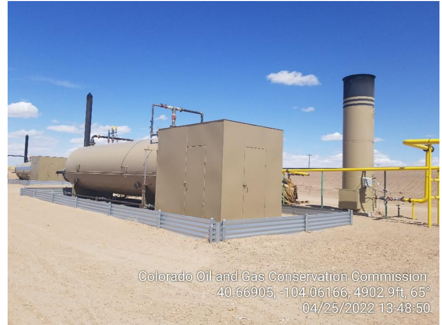
Photo 4 – Separator and ECD
