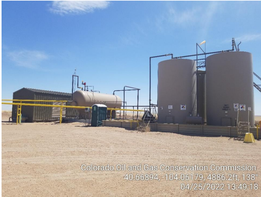
Photo 5 – Tank Battery and LACT
