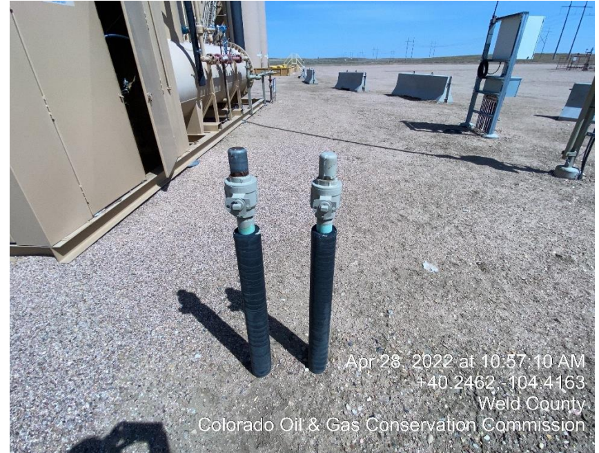
Photo #4 Unmarked Risers
