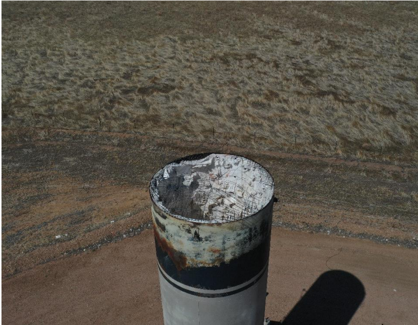
Photo #3 Missing Bird Protector
