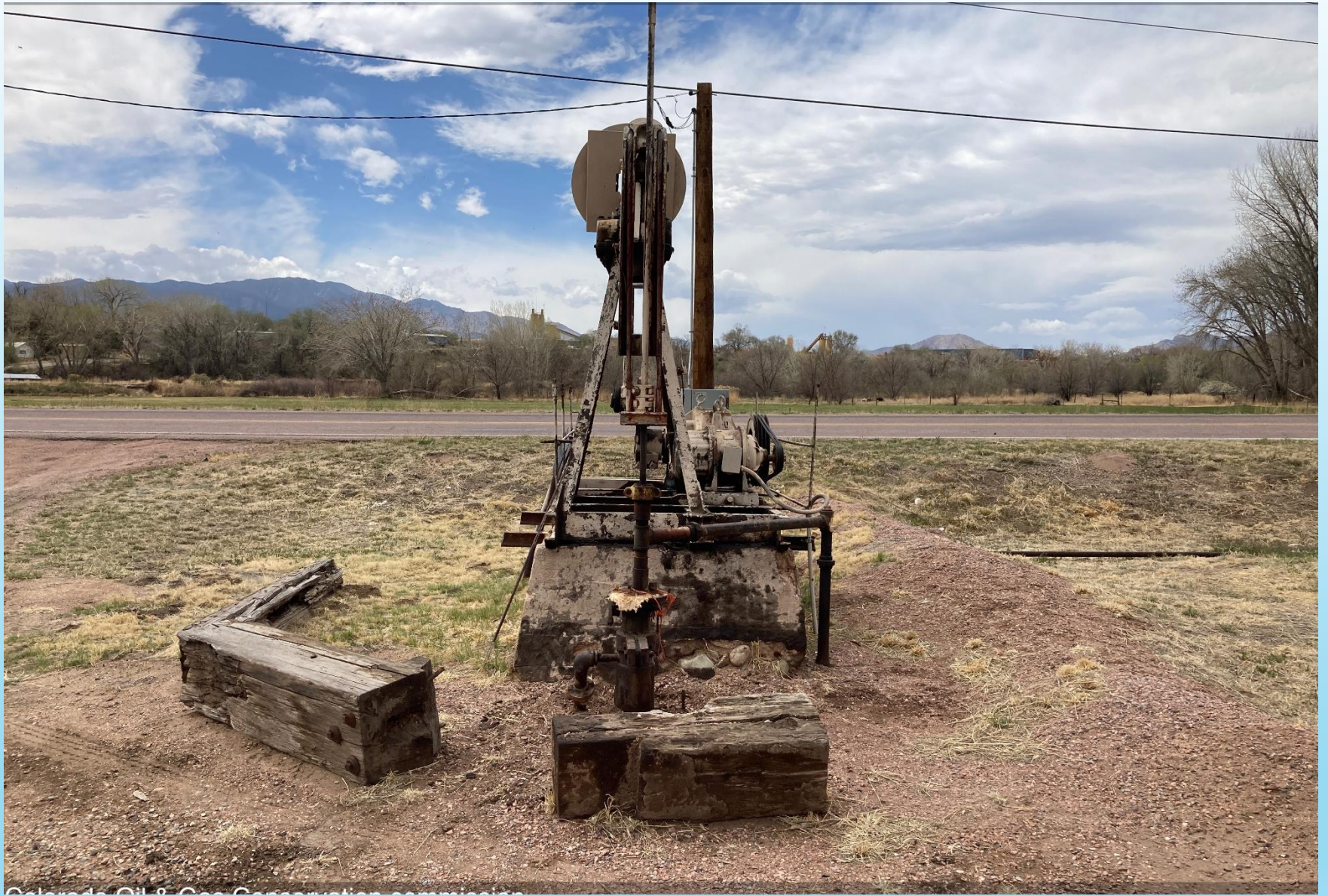
PHOTO 3: WELLHEAD AND EQUIPMENT
