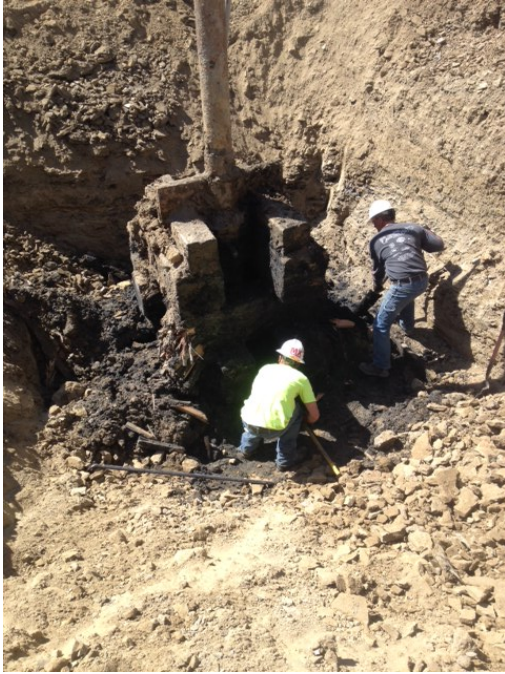
Figure 1: Well Drilled in 1933; Images from Excavation during P&A Operations
