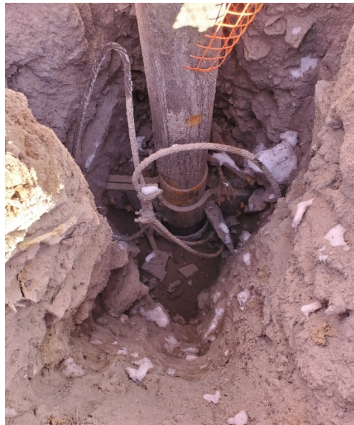
Figure 3: F Wilson #3 Casing Clamps, Hiawatha Field, CO
