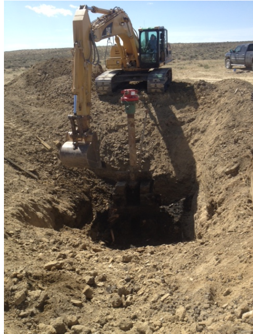
Figure 1: Well Drilled in 1933; Images from Excavation during P&A Operations
