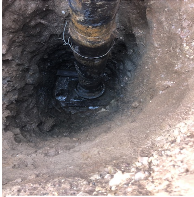
Figure 4: BW Musser #1 8-5/8" Casing Landed on top of 13-3/8", Powder Wash Field, CO
