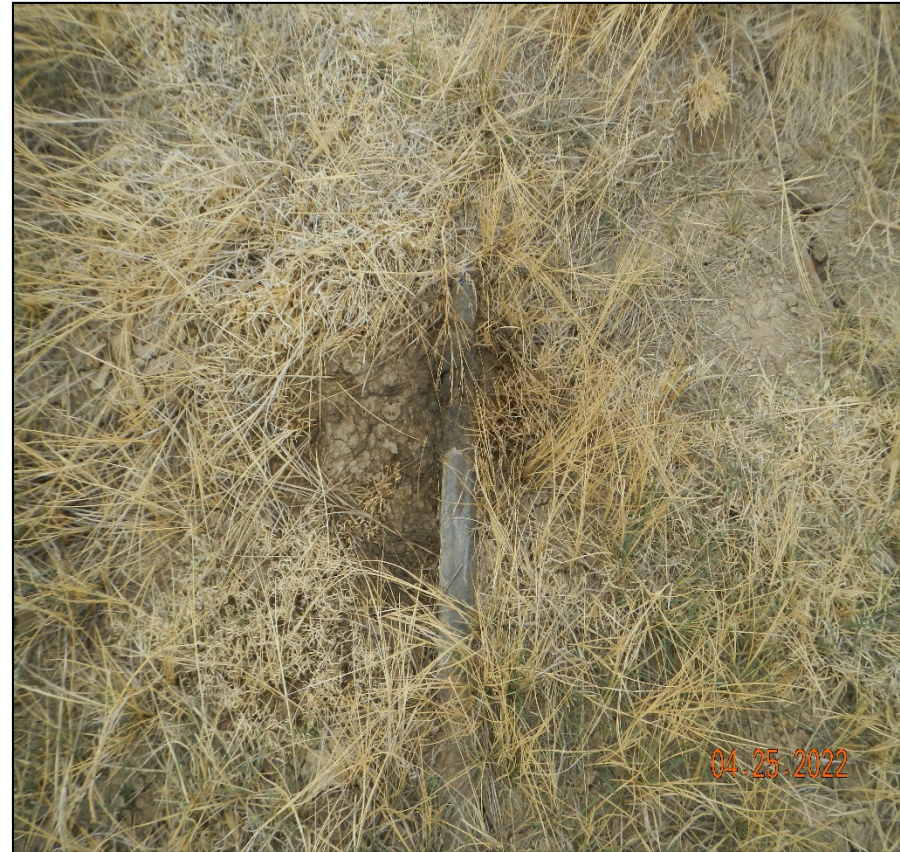
Photo 7. The impacted soils need to be cleaned up and the pipe inspected.
