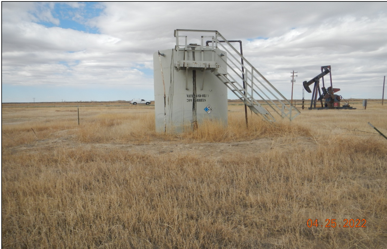
Photo 1. Facing toward the tank battery. The area inside the berm needs to be kept free of vegetation. The fence around the tank needs to be repaired to prevent livestock entry. The berm around the tank needs to be rebuilt to contain a spill.
