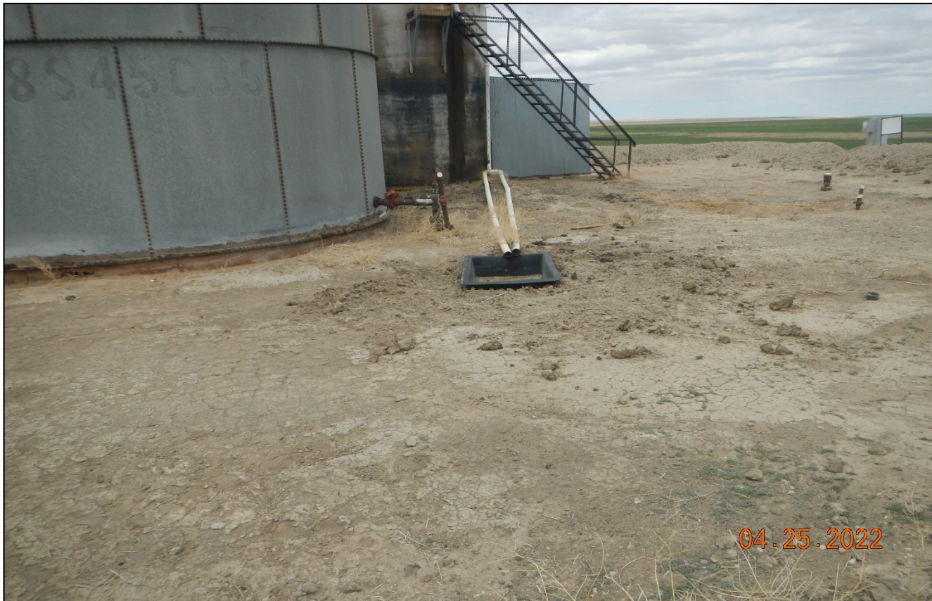
Photo 4. Oil waste has been cleaned out at the pipe outlet and a plastic tub was added to control spill. The tub will need to be monitored and cleaned out if it fills with oily waste.
