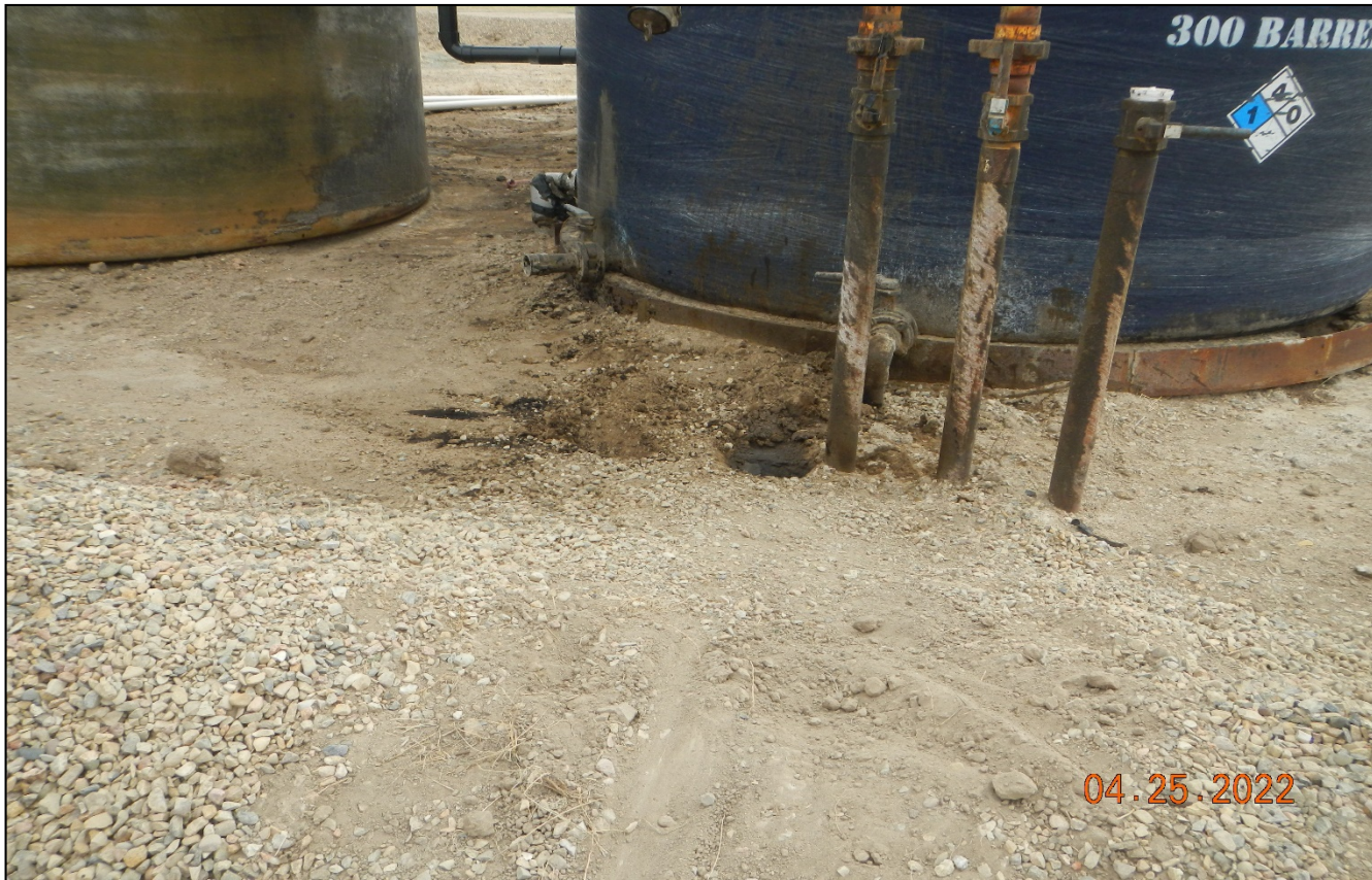
Photo 2. There is still oil stained soils that need to be cleaned up.
