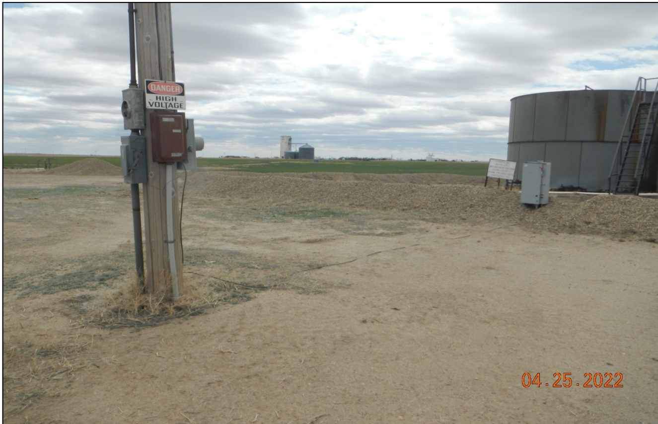
Photo 3. The electric box lid has been closed and wired. The electric cable on the ground is still a safety concern and needs to be covered and protected.
