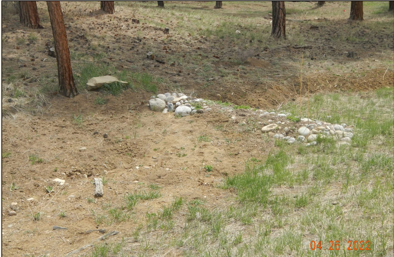
Photo 3. View of cobble BMP within the northeastern project area that is full of sediment and needs maintenance.
