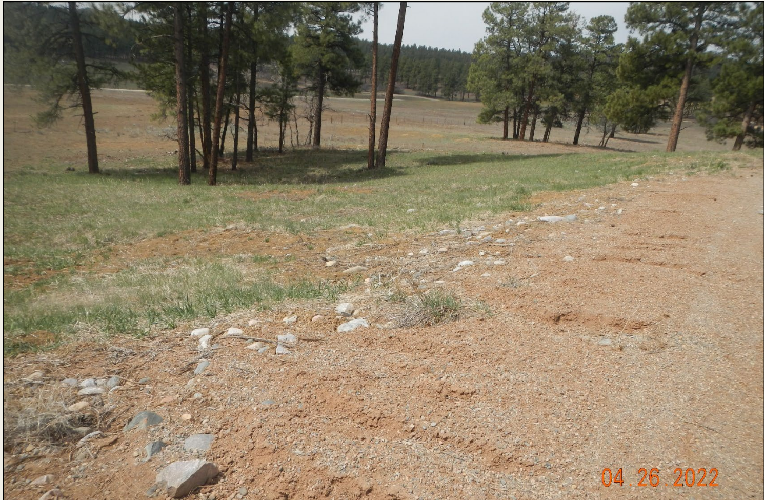
Photo 3. View of erosional rilling where concentrated stormwater flows off of the edge of the working area.
