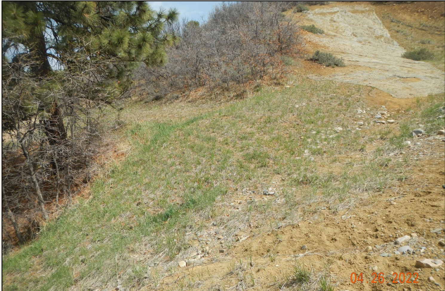
Photo 3. View of the northwestern project area facing eastward. Straw blanket needs maintenance.
