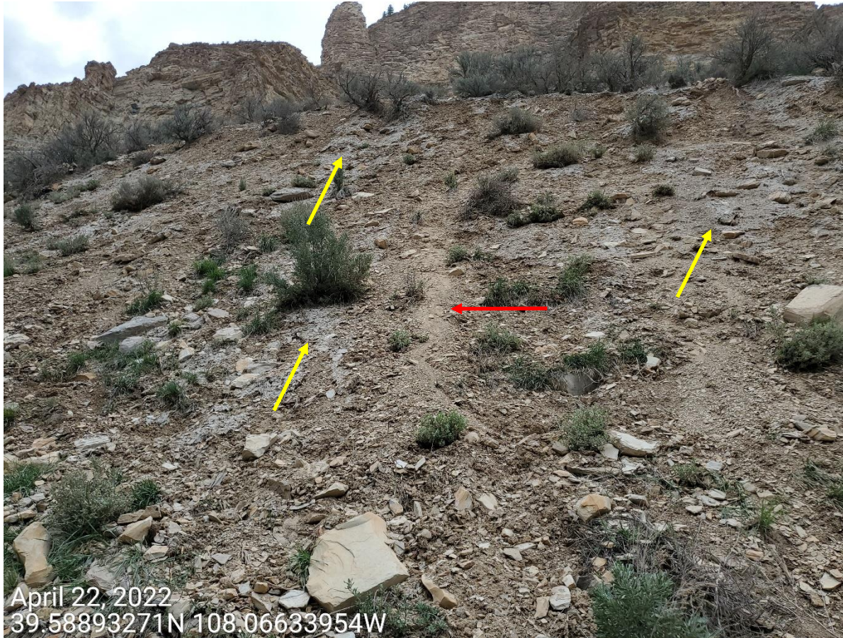
Photo 3: Photo taken from the northern interim areas of the Location. Photo example showing hydromulch (yellow arrow) that appears to have been implemented by Operator; BMP has not been maintained in a proper functioning condition to minimize erosion, degradation, and to stabilize the slopes; erosion, degradation and stabilization issues have persisted (red arrow).
