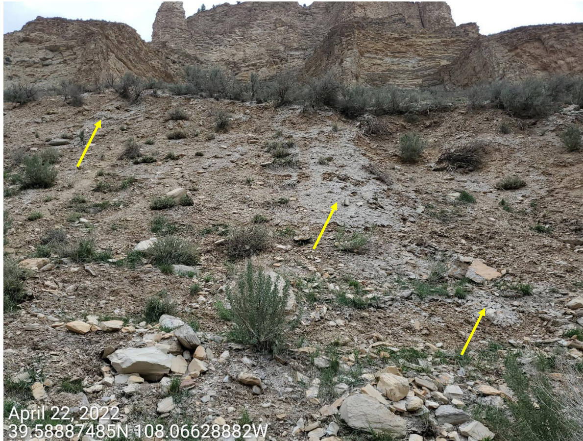
Photo 2: Photo taken from the northern interim areas of the Location. Photo example showing hydromulch (yellow arrow) that appears to have been implemented by Operator; BMP has not been maintained in a proper functioning condition to minimize erosion, degradation, and to stabilize the slopes; erosion, degradation and stabilization issues have persisted.
