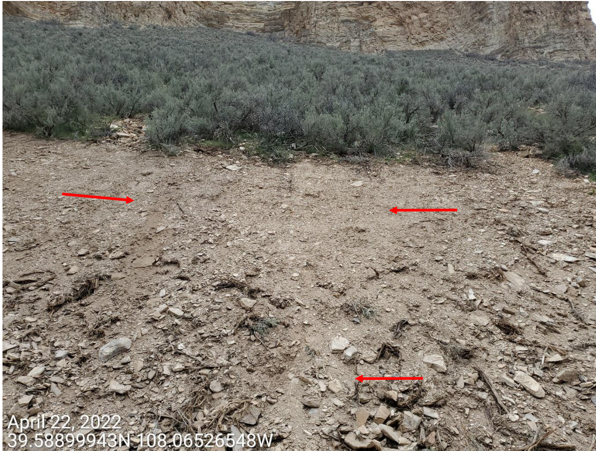
Photo 8: Photo taken from the stormwater diversion ditch along the north end of the Location. Photo example showing BMPs along slopes are missing or insufficient to minimize erosion, degradation, and to stabilize the slopes of the ditch; erosion, degradation and stabilization issues have persisted.
