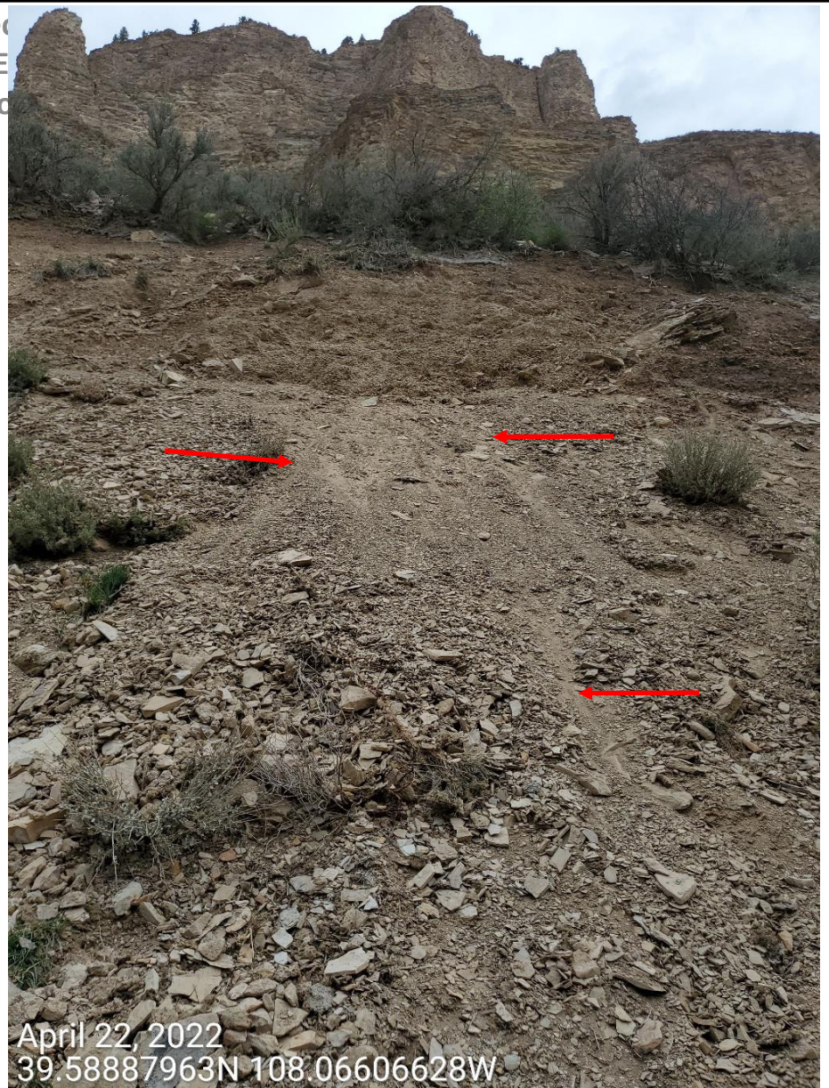
Photo 6: Photo taken from the northern interim areas of the Location. Photo example showing BMPs along slopes have not been maintained in a proper functioning condition to minimize erosion, degradation, and to stabilize the slopes; erosion, degradation and stabilization issues have persisted.
