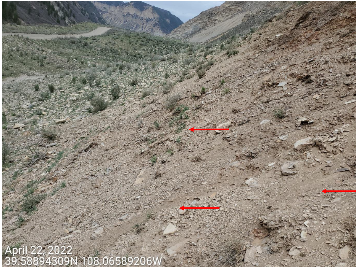
Photo 5: Photo taken from the northern interim areas of the Location. Photo example showing BMPs along slopes have not been maintained in a proper functioning condition to minimize erosion, degradation, and to stabilize the slopes; erosion, degradation and stabilization issues have persisted.
