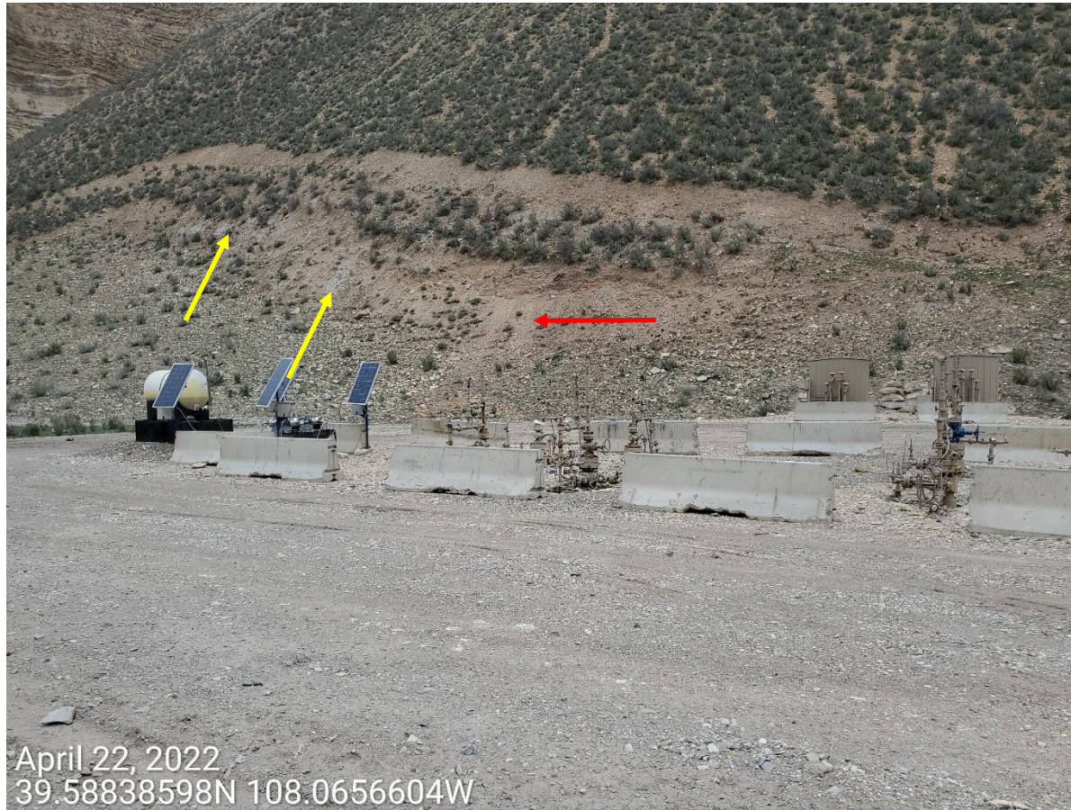
Photo 1: Photo taken from the location, facing north. Photo provides overview of the northern interim areas of the Location and the perimeter stormwater ditch. Operator appears to have implemented hydromulch (yellow arrow) at slopes, however BMP has not been maintained in a proper functioning condition to minimize erosion, degradation, and to stabilize the slopes; erosion and degradation to the slopes have persisted (red arrow example).
