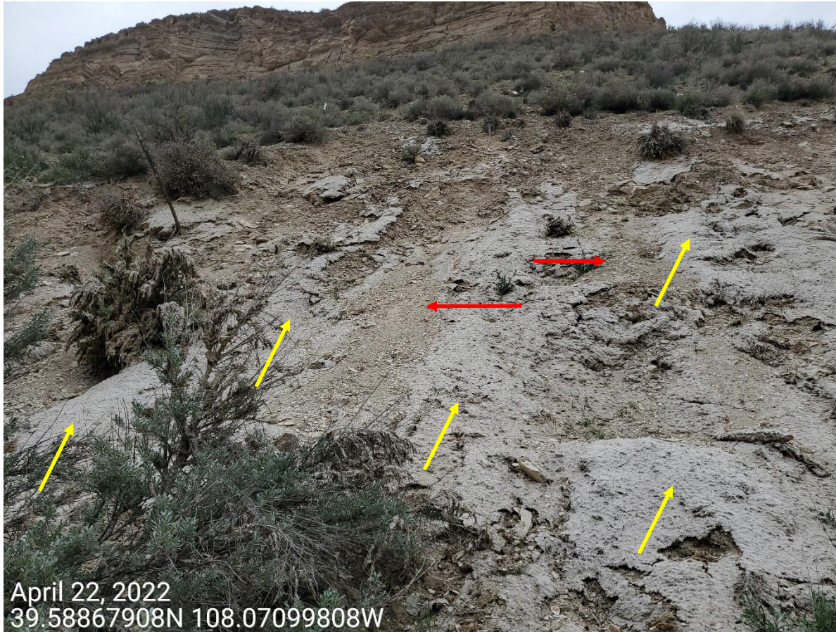
Photo 4: Photo taken from the disturbed slopes on the north end of the Location. Photo example showing hydromulch (yellow arrow) implemented by Operator has not been maintained in a proper functioning condition to minimize erosion, degradation, and to stabilize the slopes; erosion and degradation to the slopes have persisted. Red arrow shows areas where soils have eroded and covered sections of the hydromulch
