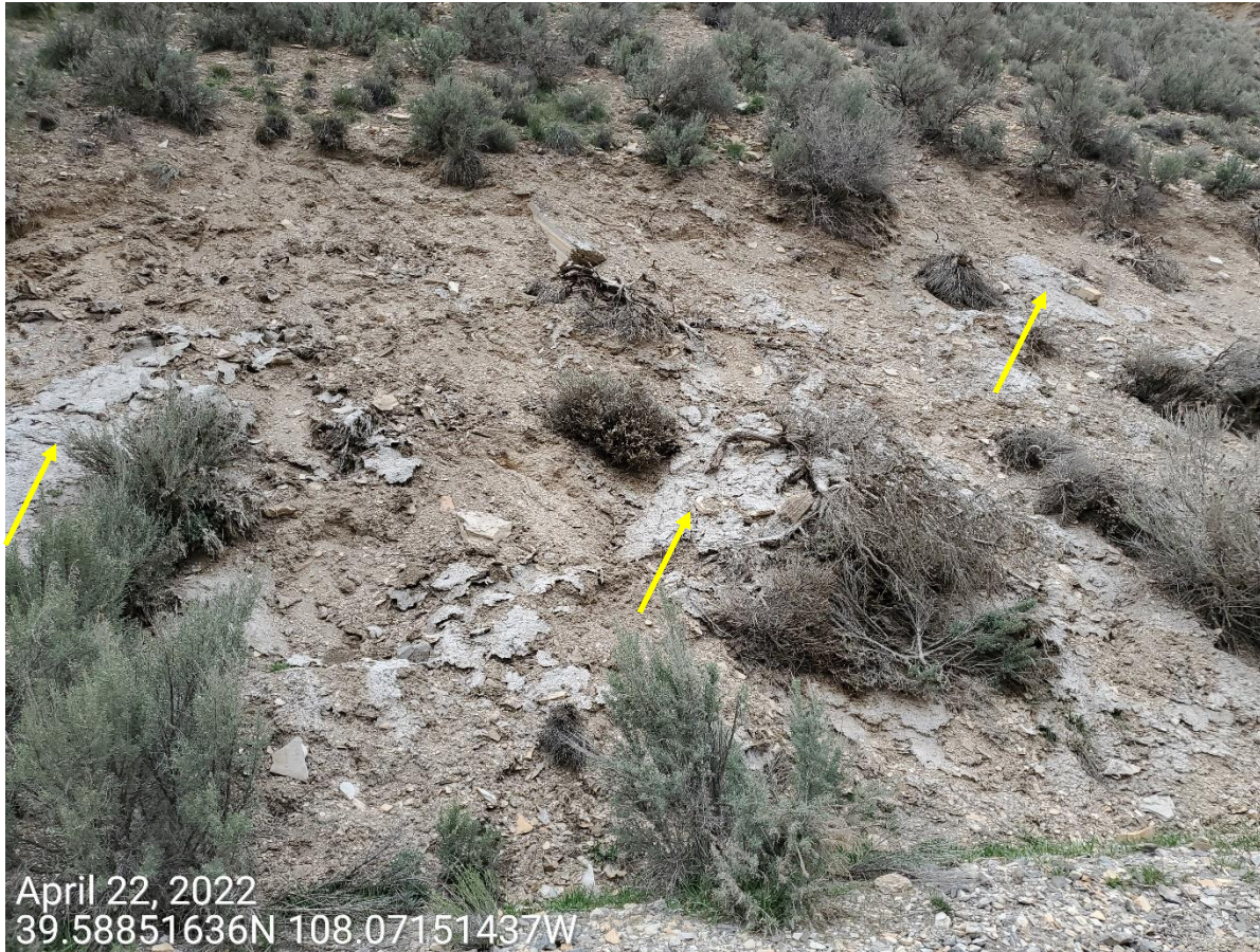
Photo 1: Photo taken from the disturbed slopes on the north end of the Location. Photo example showing hydromulch (yellow arrow) implemented by Operator has not been maintained in a proper functioning condition to minimize erosion, degradation, and to stabilize the slopes; erosion and degradation to the slopes have persisted.
