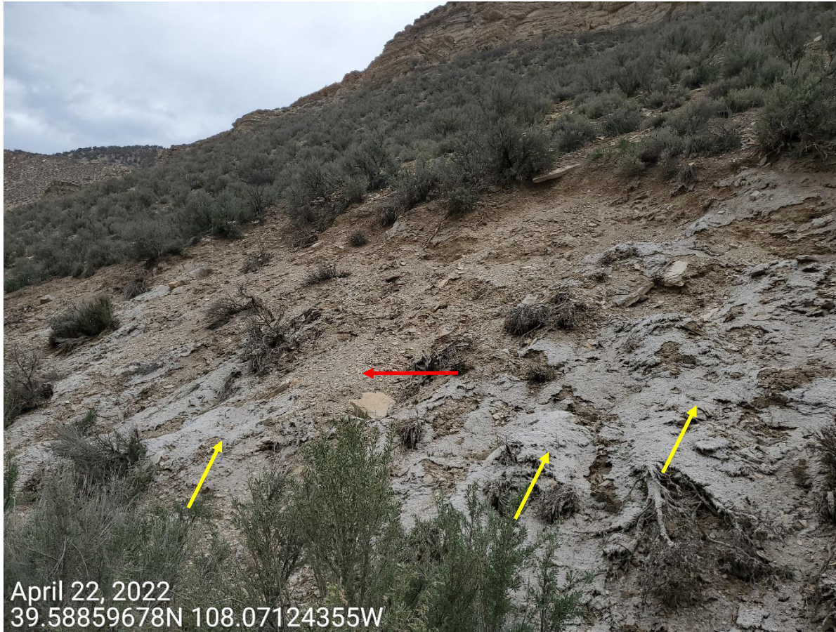
Photo 3: Photo taken from the disturbed slopes on the north end of the Location. Photo example showing hydromulch (yellow arrow) implemented by Operator has not been maintained in a proper functioning condition to minimize erosion, degradation, and to stabilize the slopes; erosion and degradation to the slopes have persisted. Red arrow shows areas where soils have eroded and covered sections of the hydromulch
