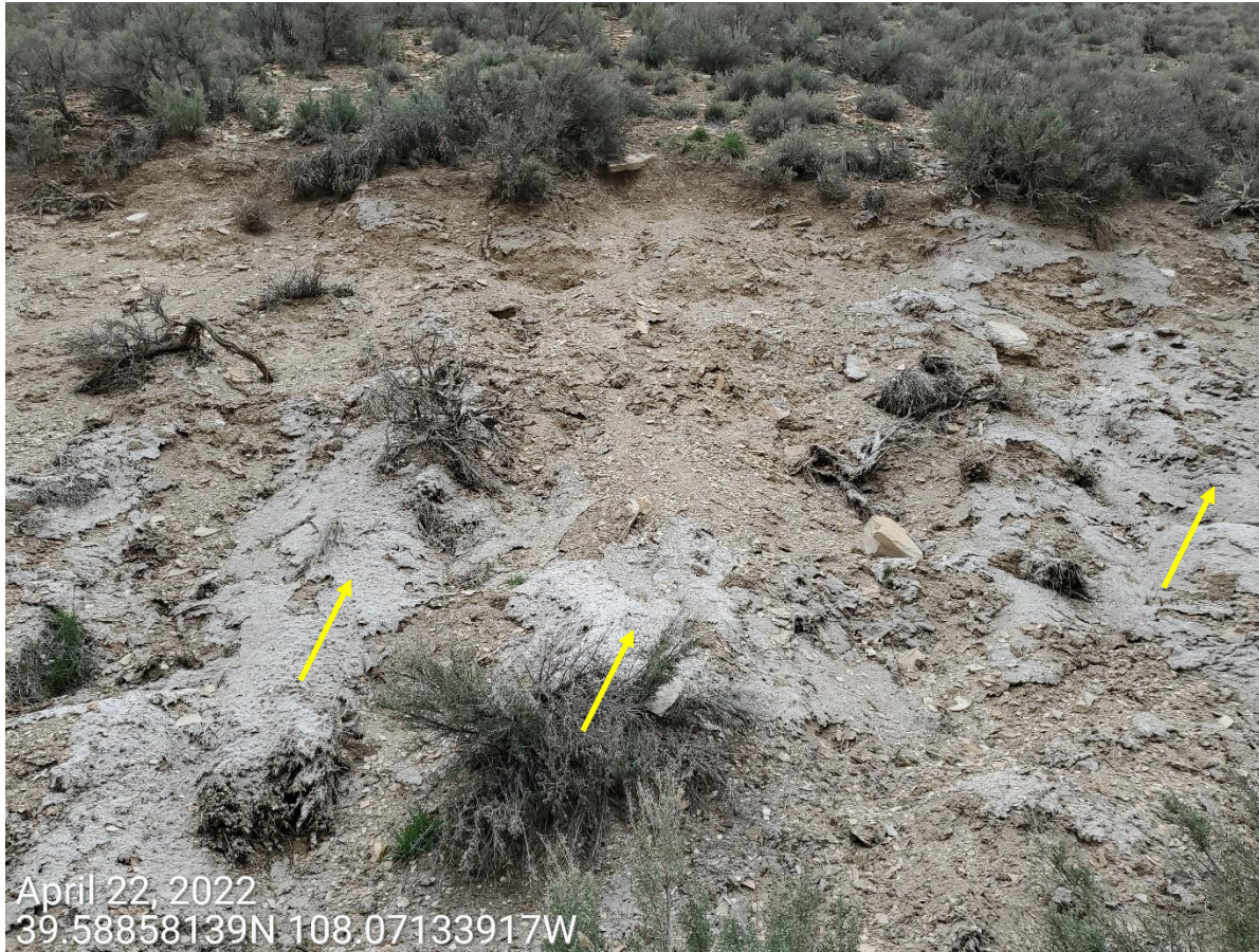
Photo 2: Photo taken from the disturbed slopes on the north end of the Location. Photo example showing hydromulch (yellow arrow) implemented by Operator has not been maintained in a proper functioning condition to minimize erosion, degradation, and to stabilize the slopes; erosion and degradation to the slopes have persisted.
