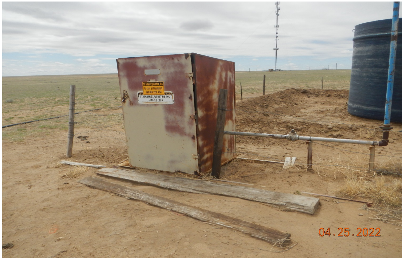
Photo 4. Sign post is not sufficient per 605.a. No other well sign was observed.
