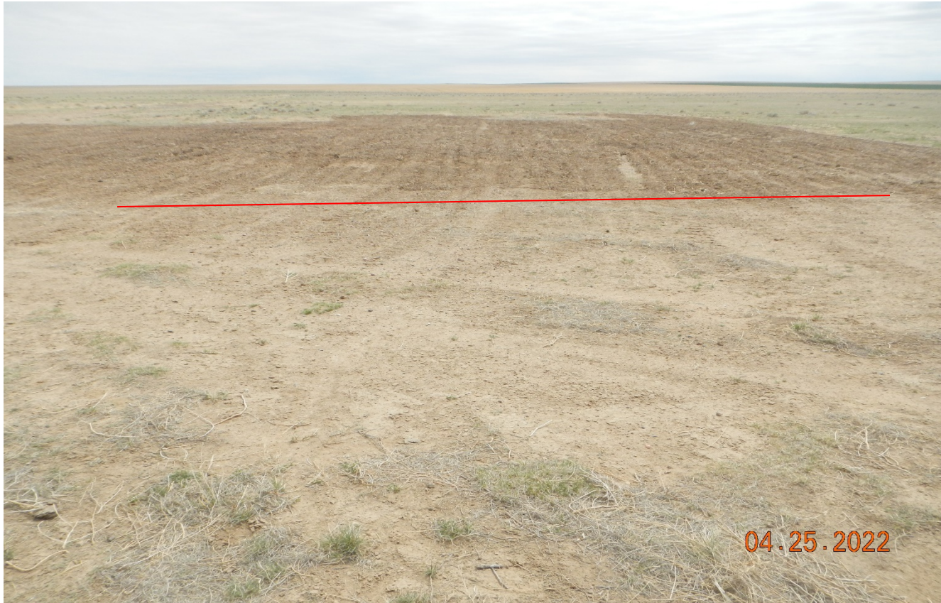
Photo 6. Facing east toward the location. The entire disturbed location was not properly decompacted. Soils were ripped above red line but not below.
