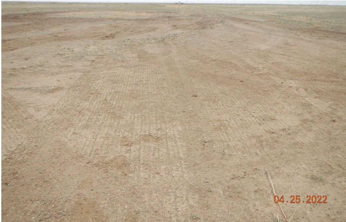
Photo 13. Soils remain compacted in areas of the location. Cross ripping of soils must be performed to at least 18 inches along with tilling to establish a proper seedbed.
