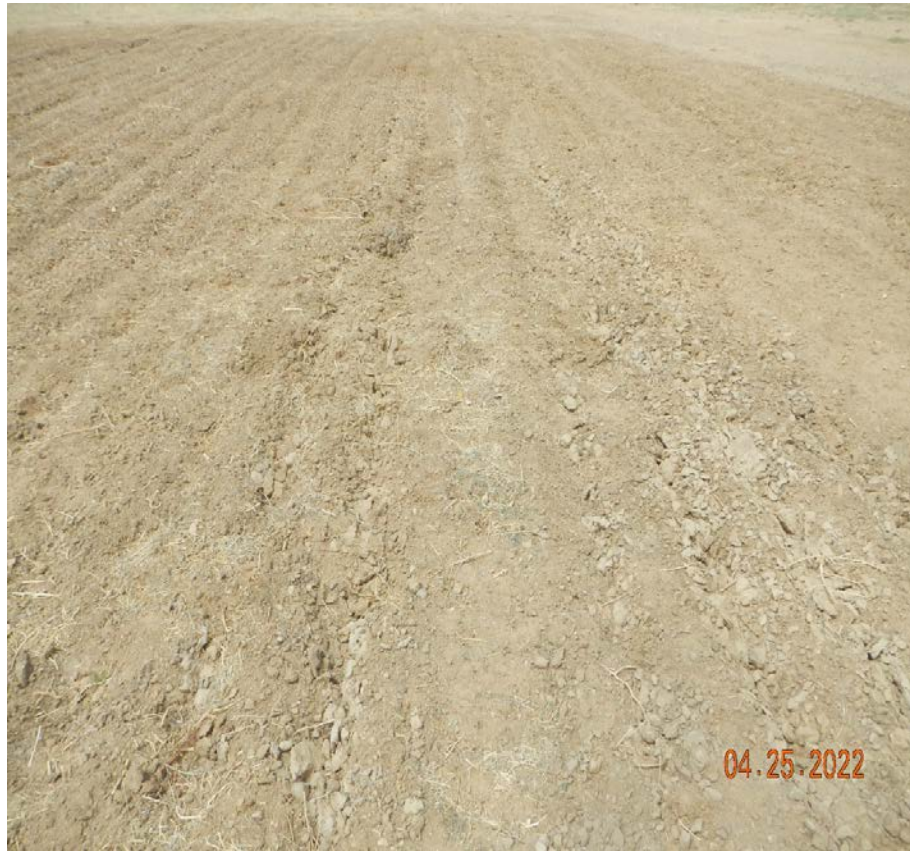
Photo 4. Soils have been ripped one direction. 1003.c. requires decompaction by cross ripping.
