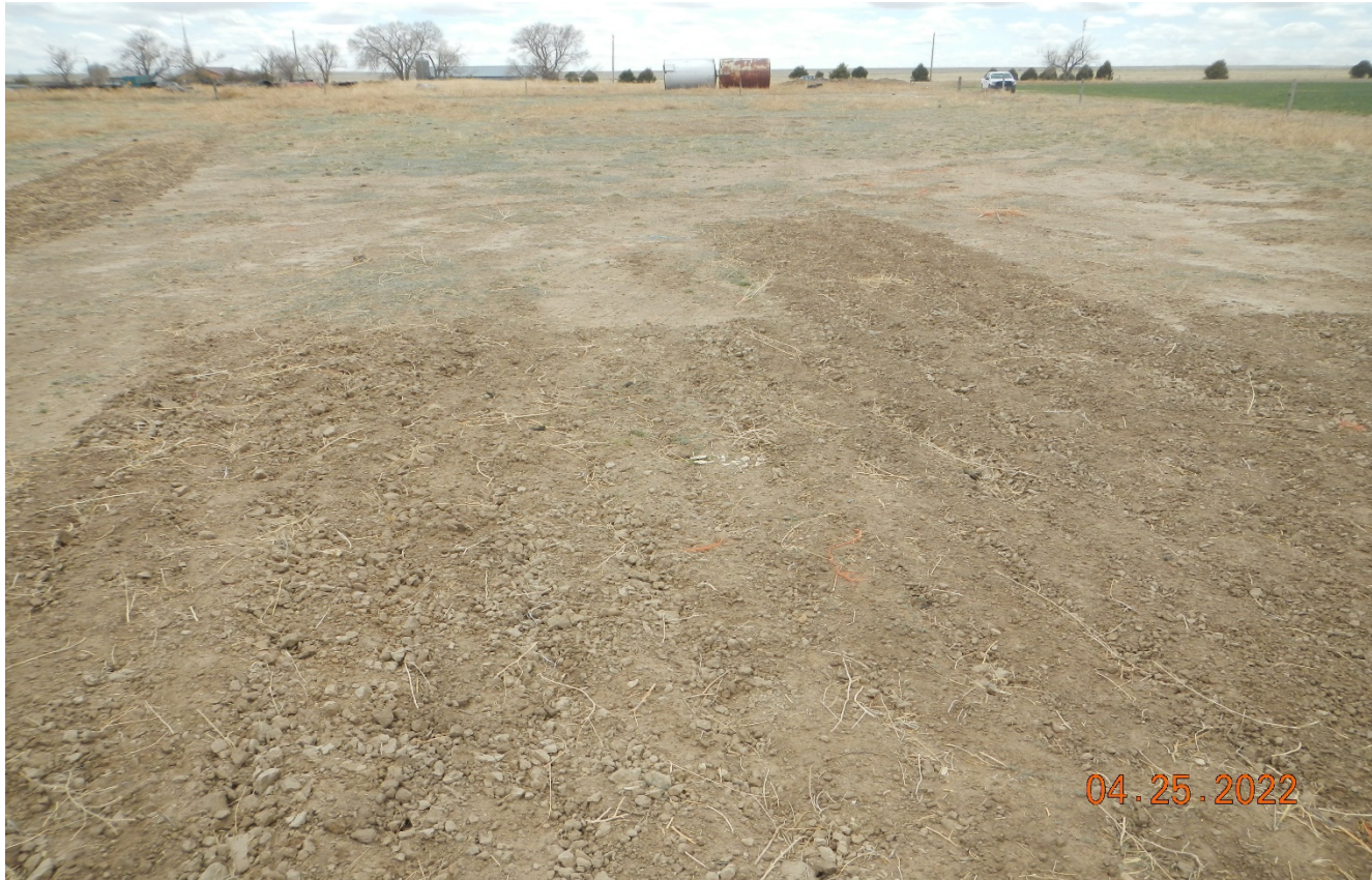
Photo 3. Facing south at the location. There are areas where soil has been decompacted and other areas that remain compacted. Unable to determine if seeding was performed (No seed observed on the soil surface).
