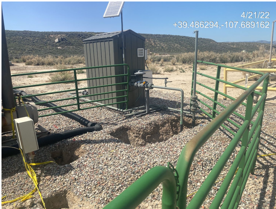
Photo 2. Photo taken from the separator at the northeast of the Location shows inadequate protection of an excavated area from entrance by wildlife, livestock or personnel.
