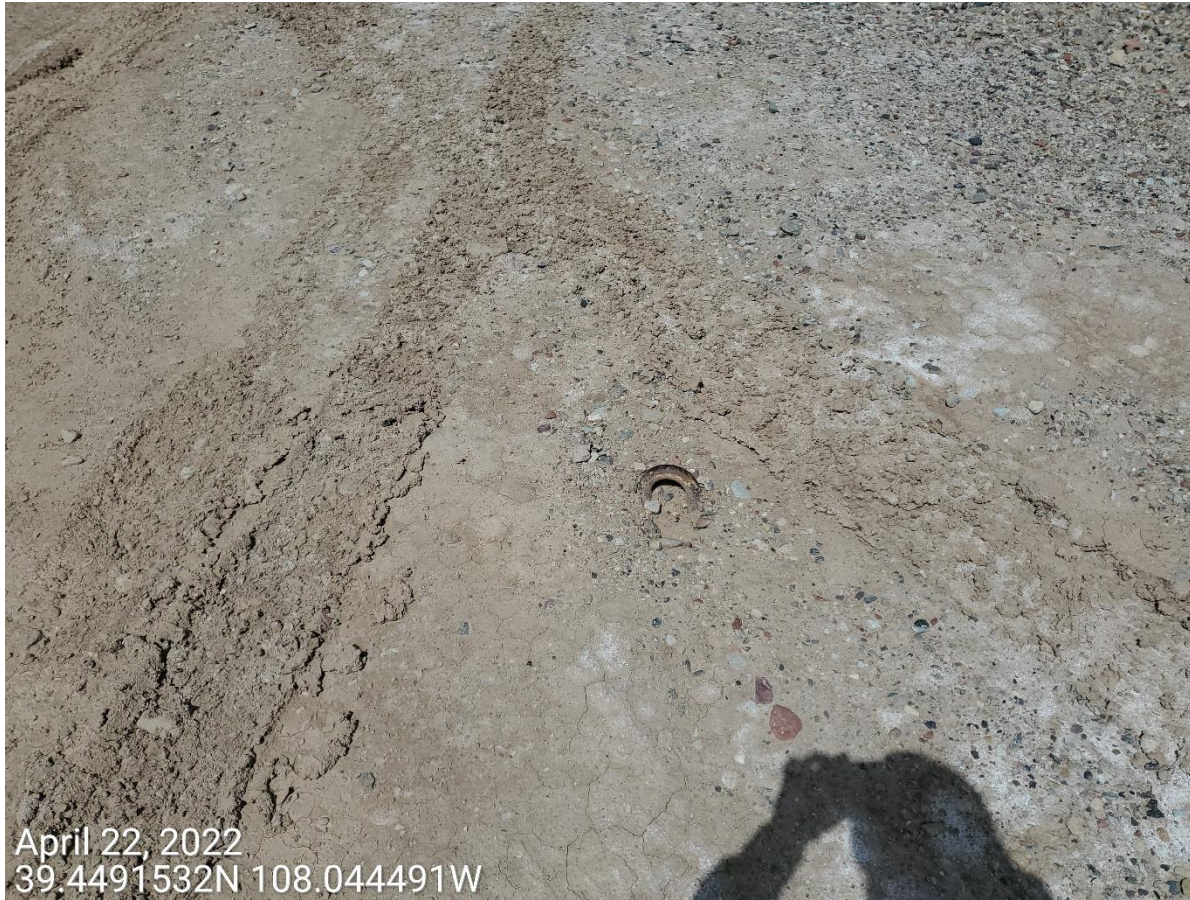
Photo 2: Photo example of unmarked anchor observed on Location.
