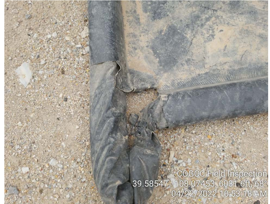
Photo #4 – Mobile separator secondary containment device in need of repair.
