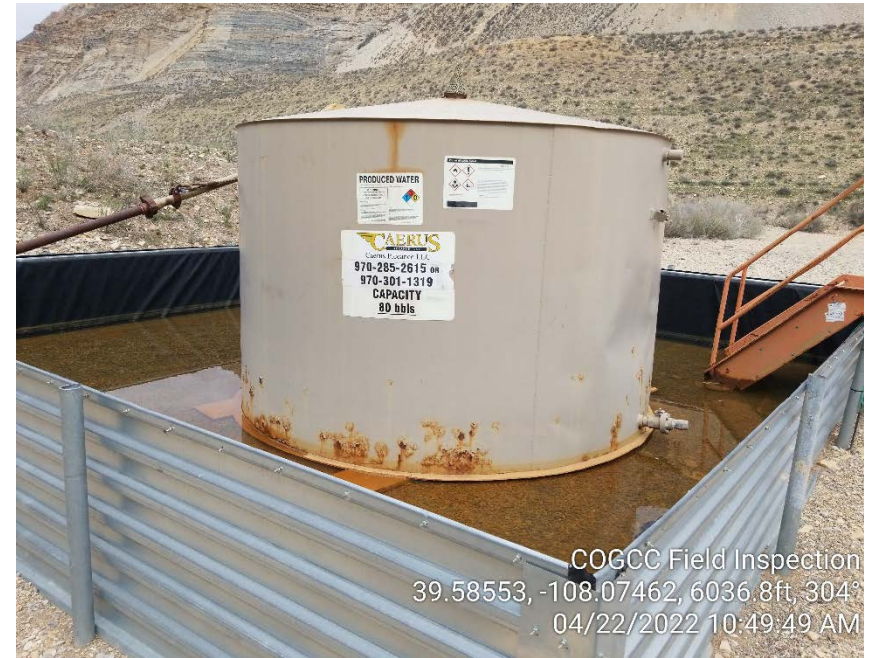
Photo #2 – 80 bbl produced water AST on west end of pad. Note that secondary containment was filled with fluids on inspection date. No hydrocarbon sheens or odors were observed on fluids during inspection.
