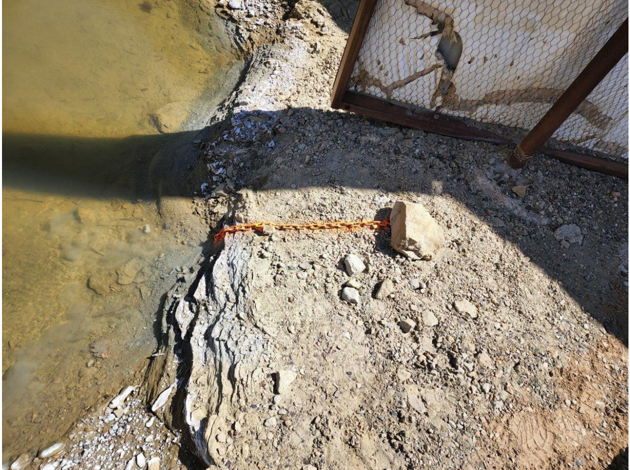
Installed Freeboard Marker per Rule 909.
