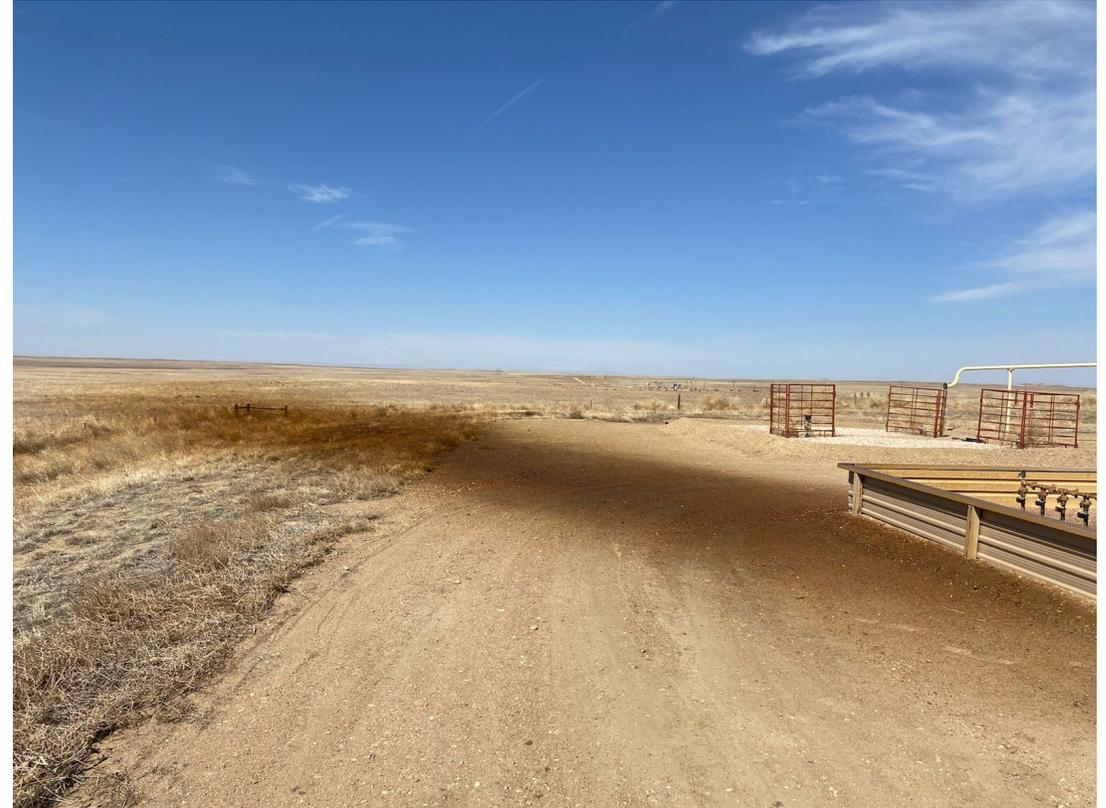
Oil release from separator to tank battery/pad surface and adjacent vegetation
