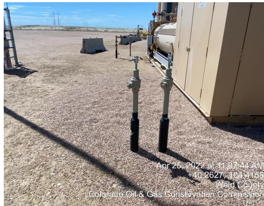
Photo #4 Unmarked Risers
