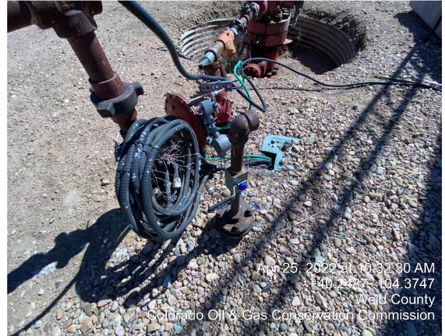
Photo #8 Unmarked Riser
