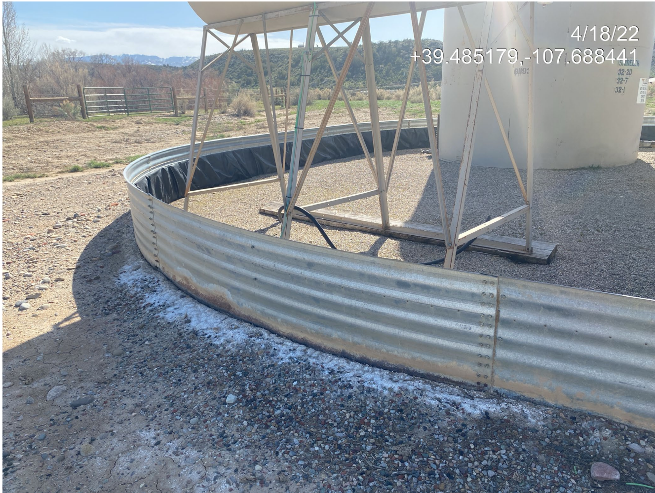
Photo 3. Photo taken from the tank battery shows salt staining outside of secondary containment along the northeast side of the tank battery. Corrosion is apparent at the base of the metal containment
