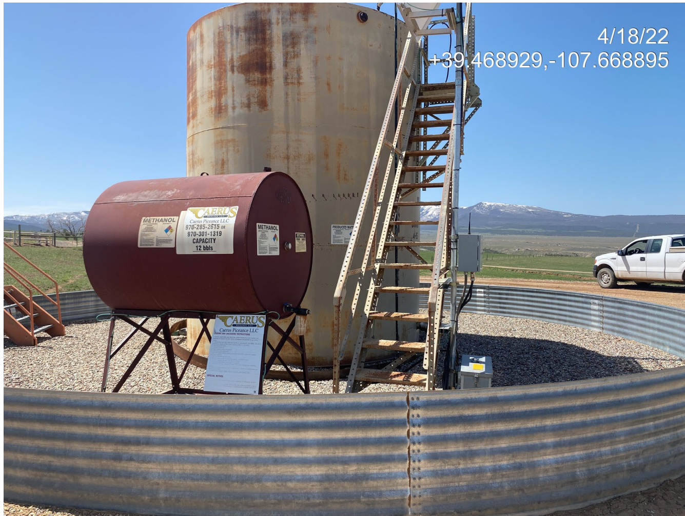
Photo 2. Photo taken from tank battery facing west shows a lack of proper signage at the tank battery.
