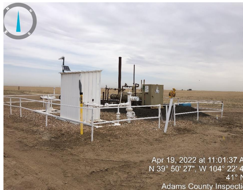
Photo # 2 Meter house & Separator.
