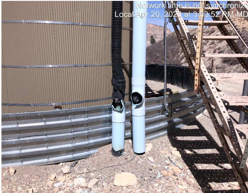
Photo #6537 Heating insulation open ended.
