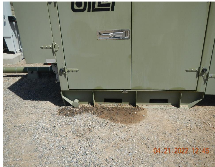
Stained soil next to OilLift pump controller.
