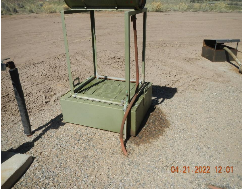
Lube oil is leaking onto the ground next to the secondary containment.
