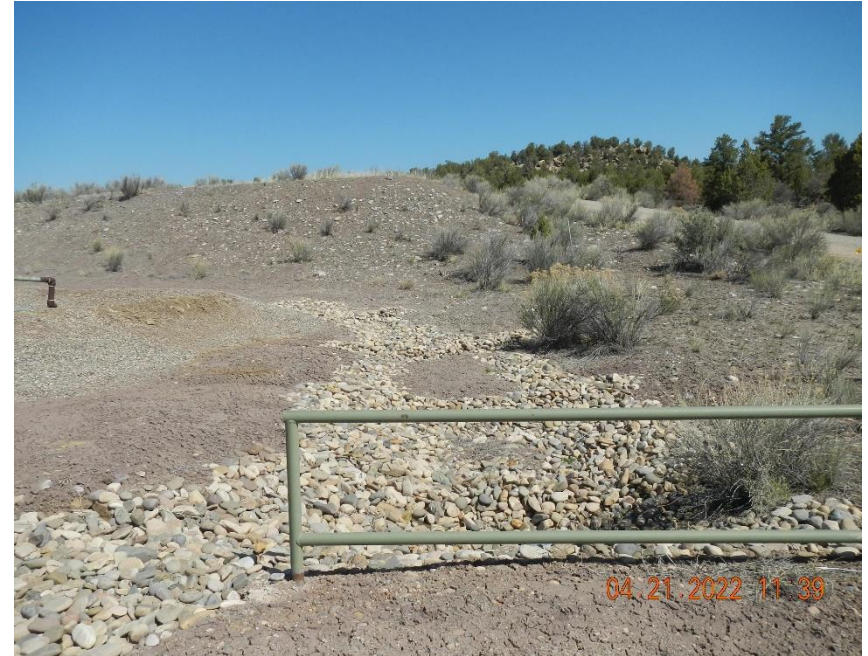
Rip rap and sediment traps along northeastern edge of the location.
