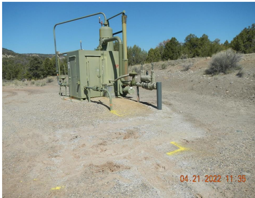
Leaking water line valve on separator resulting in Spill/Release Point ID #481990.
