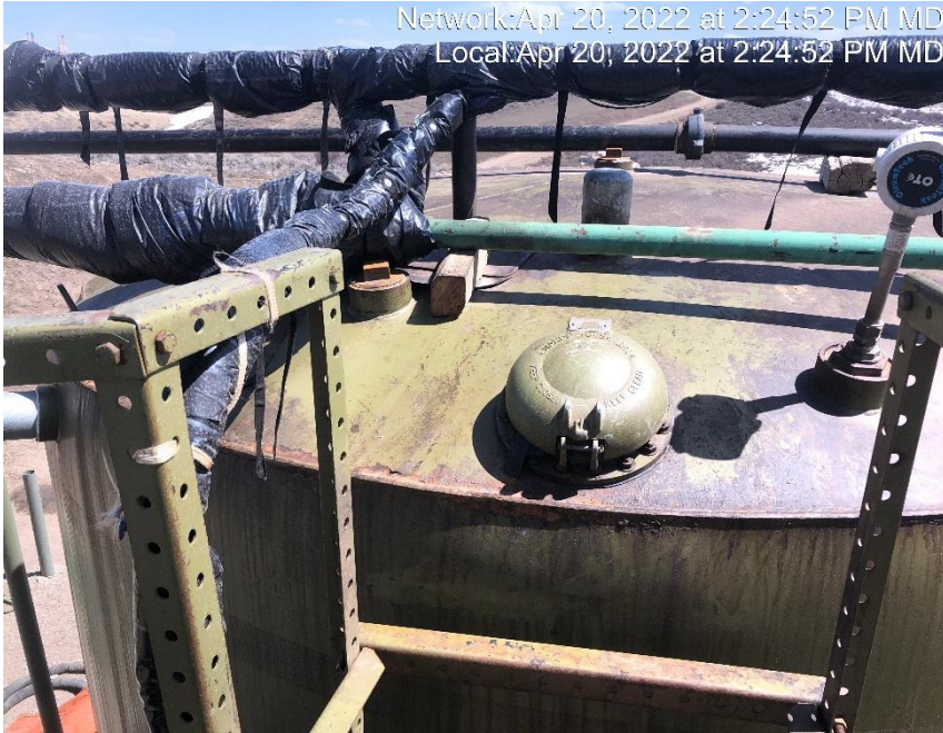
Photo #6525 Tank appears to have been over pressured and is disconnected.
