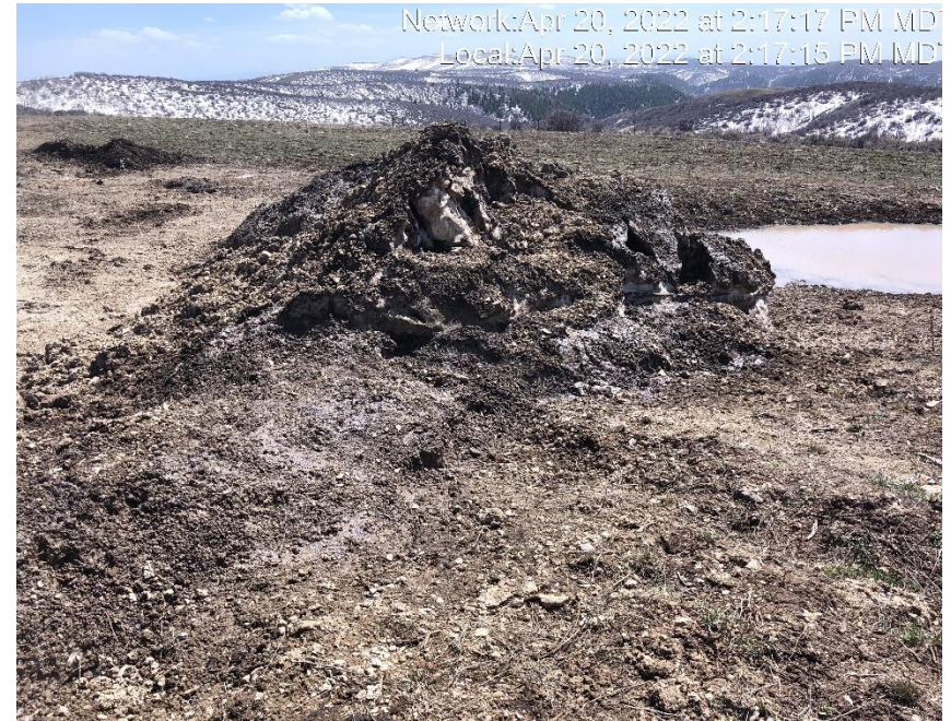
Photo #6524 Sediment has been transported on to reclaimed area.
