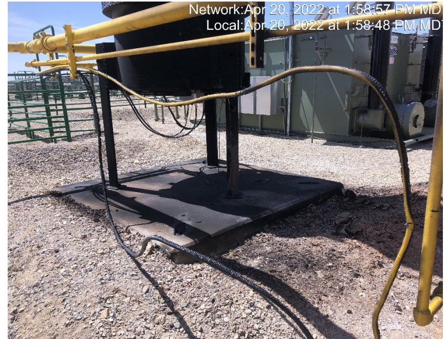
Photo #6491 Melted automation lines.
