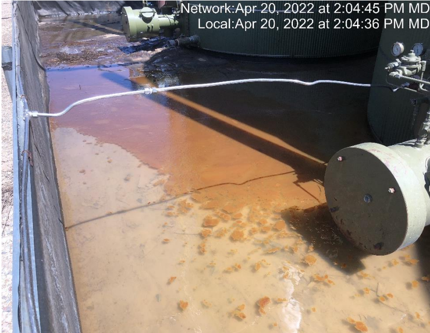
Photo #6500 Oily fluid located throughout containment.
