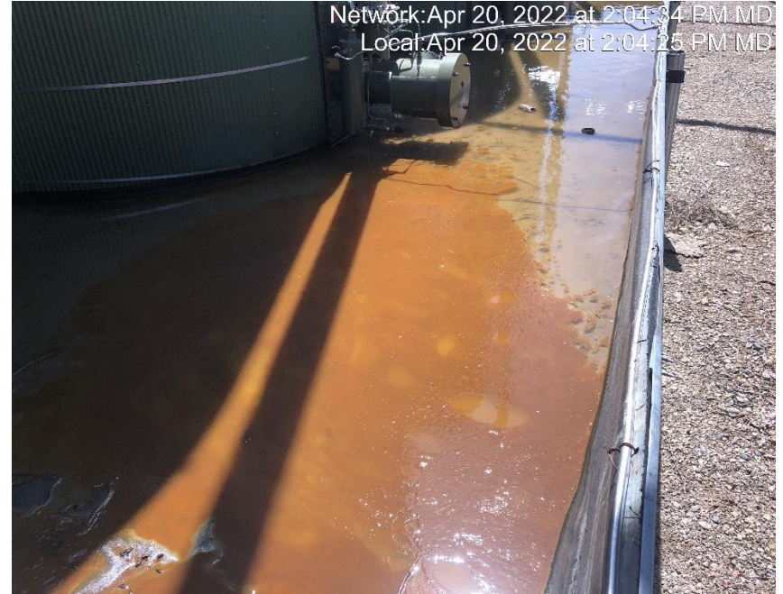
Photo #6499 Oily fluid located throughout containment.
