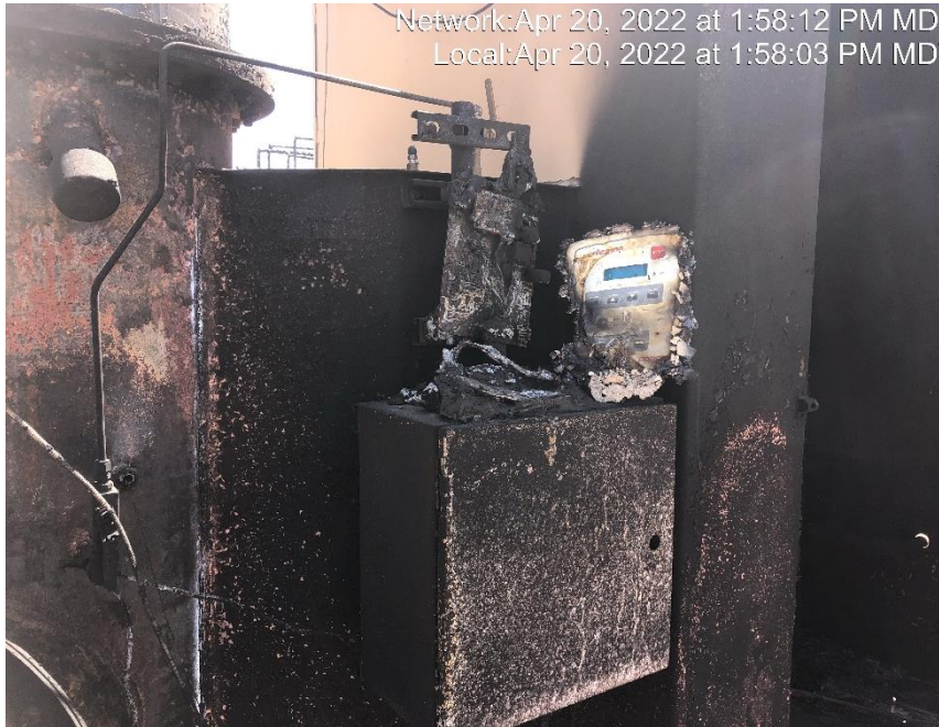
Photo #6490 Burned Pro Fire ignition controller.
