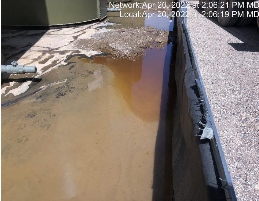
Photo #6507 Oily fluid located throughout containment.
