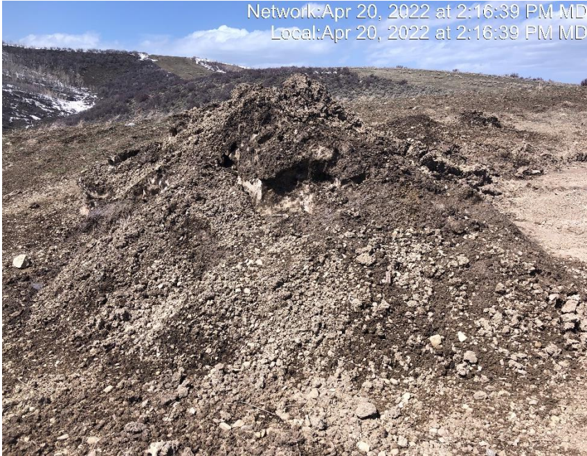
Photo #6522 Multiple piles of sediment without BMP implementation.
