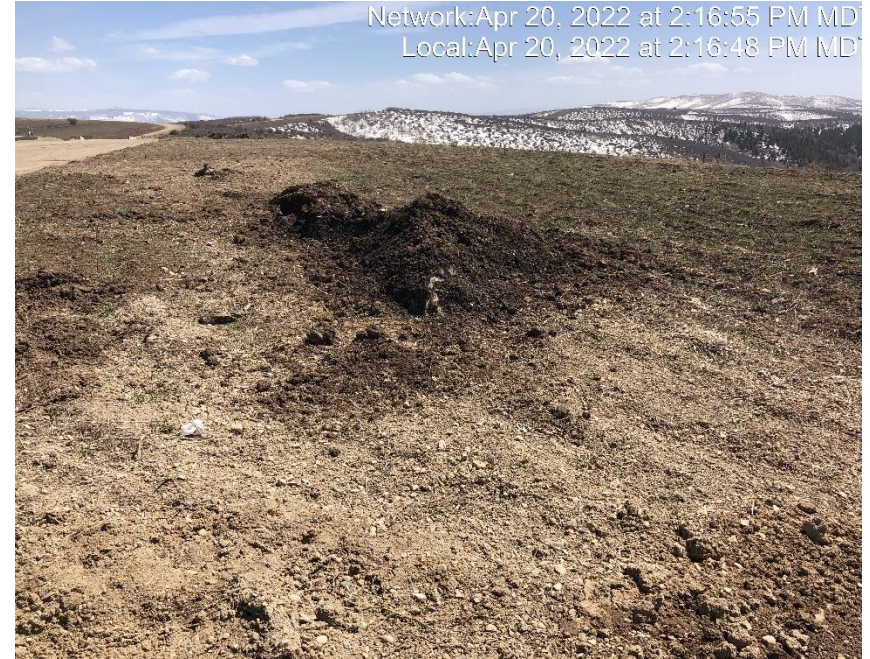
Photo #6523 Sediment has been transported on to reclaimed area.
