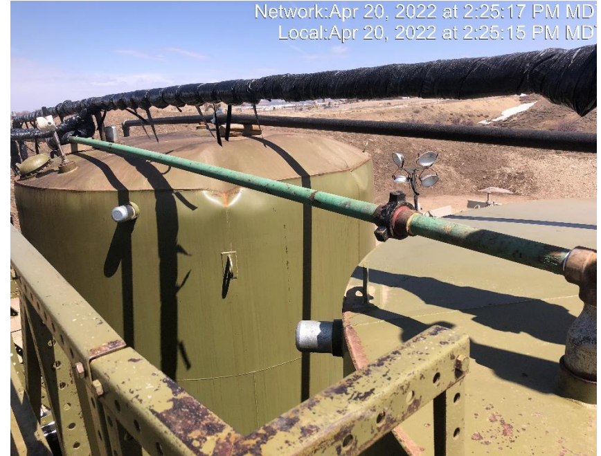
Photo #6526 Tank appears to have been over pressured and is disconnected.
