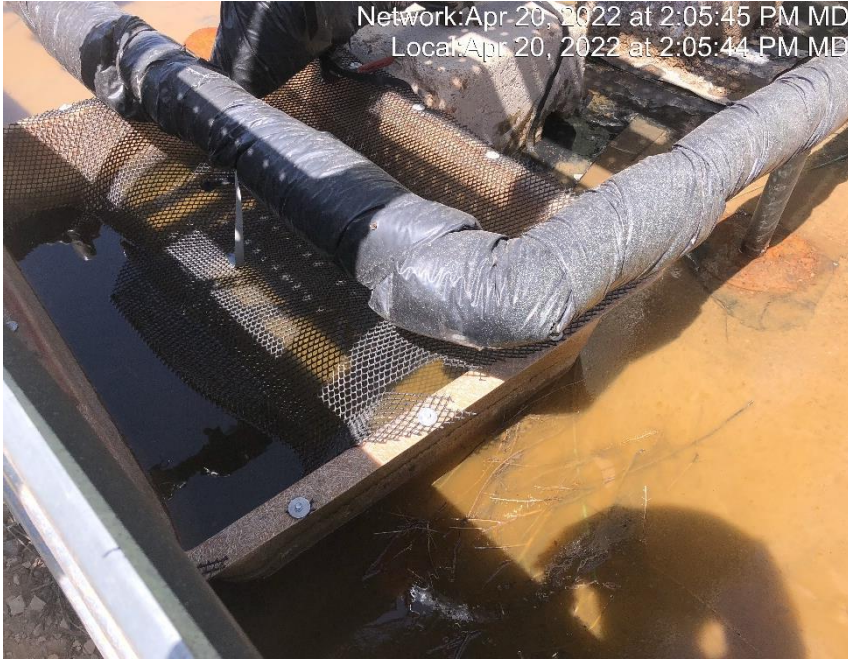
Photo #6504 Bird protector insufficient.
