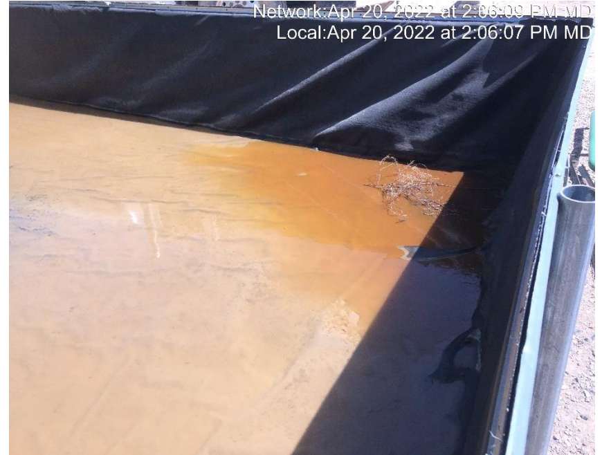
Photo #6506 Oily fluid located throughout containment.
