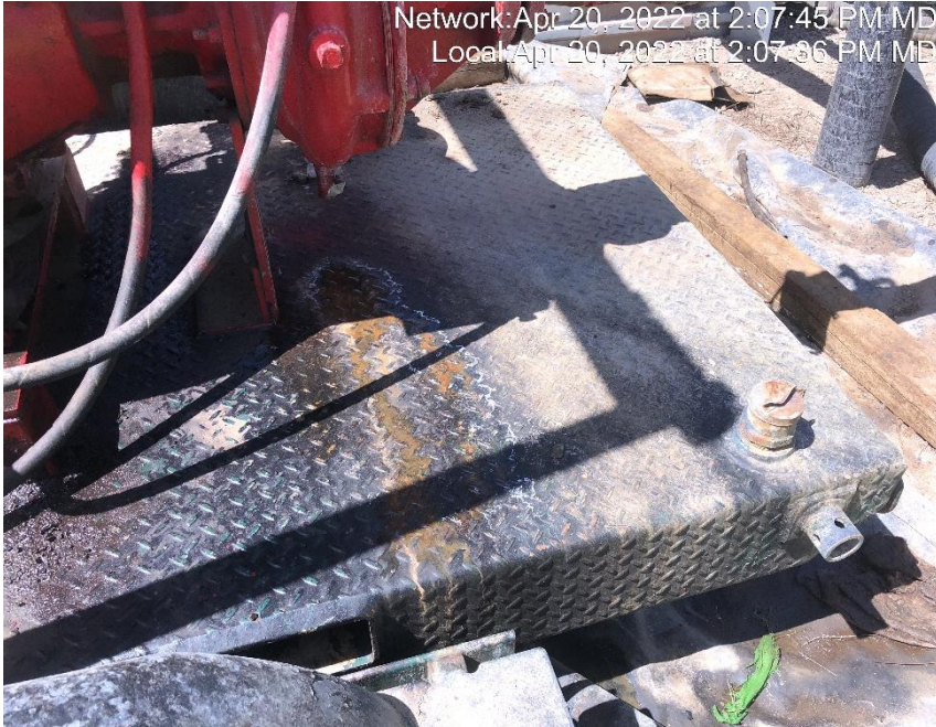
Photo #6510 Drain valve on produced water transfer pump appears to be leaking.
