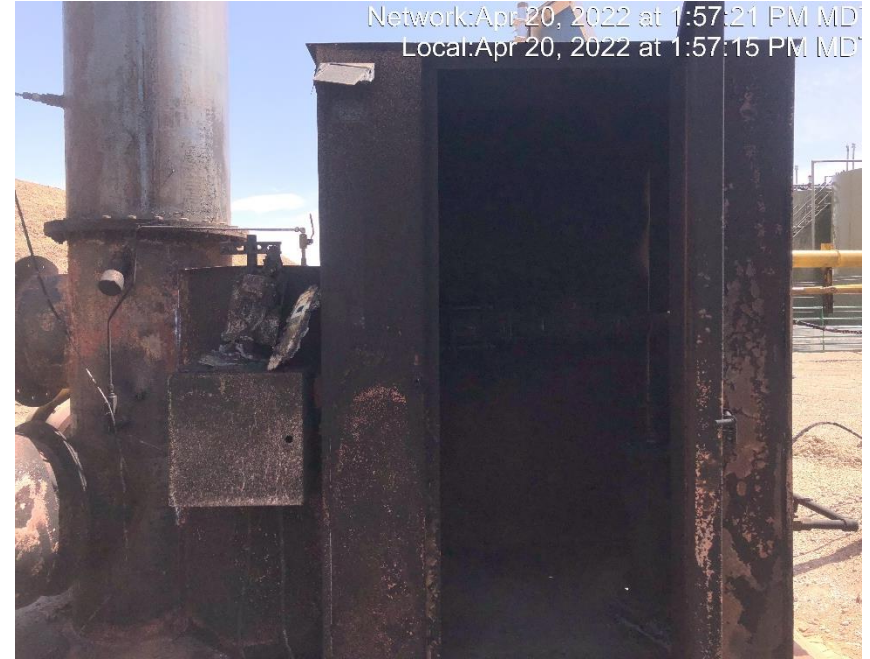
Photo #6489 combustor fire.
