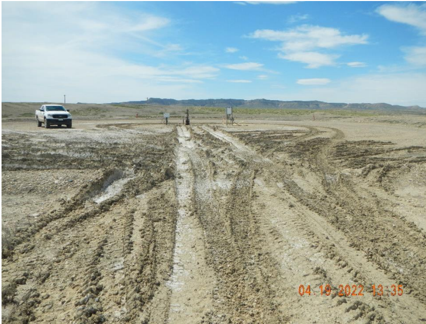
Deep ruts on location are sign of lack of compaction
