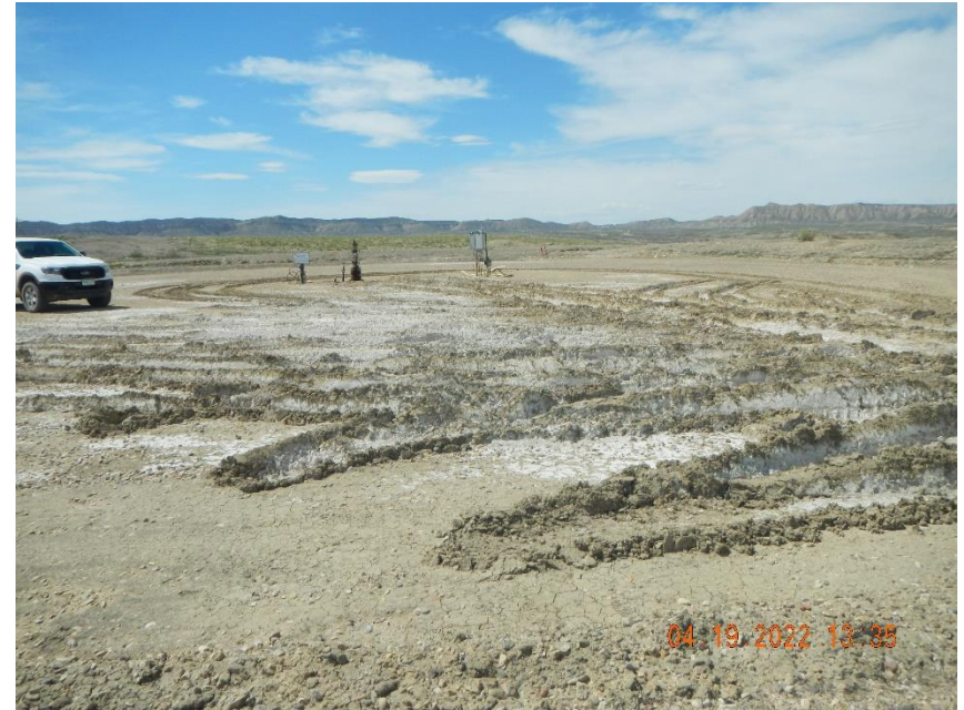
Deep ruts on location are sign of lack of compaction
