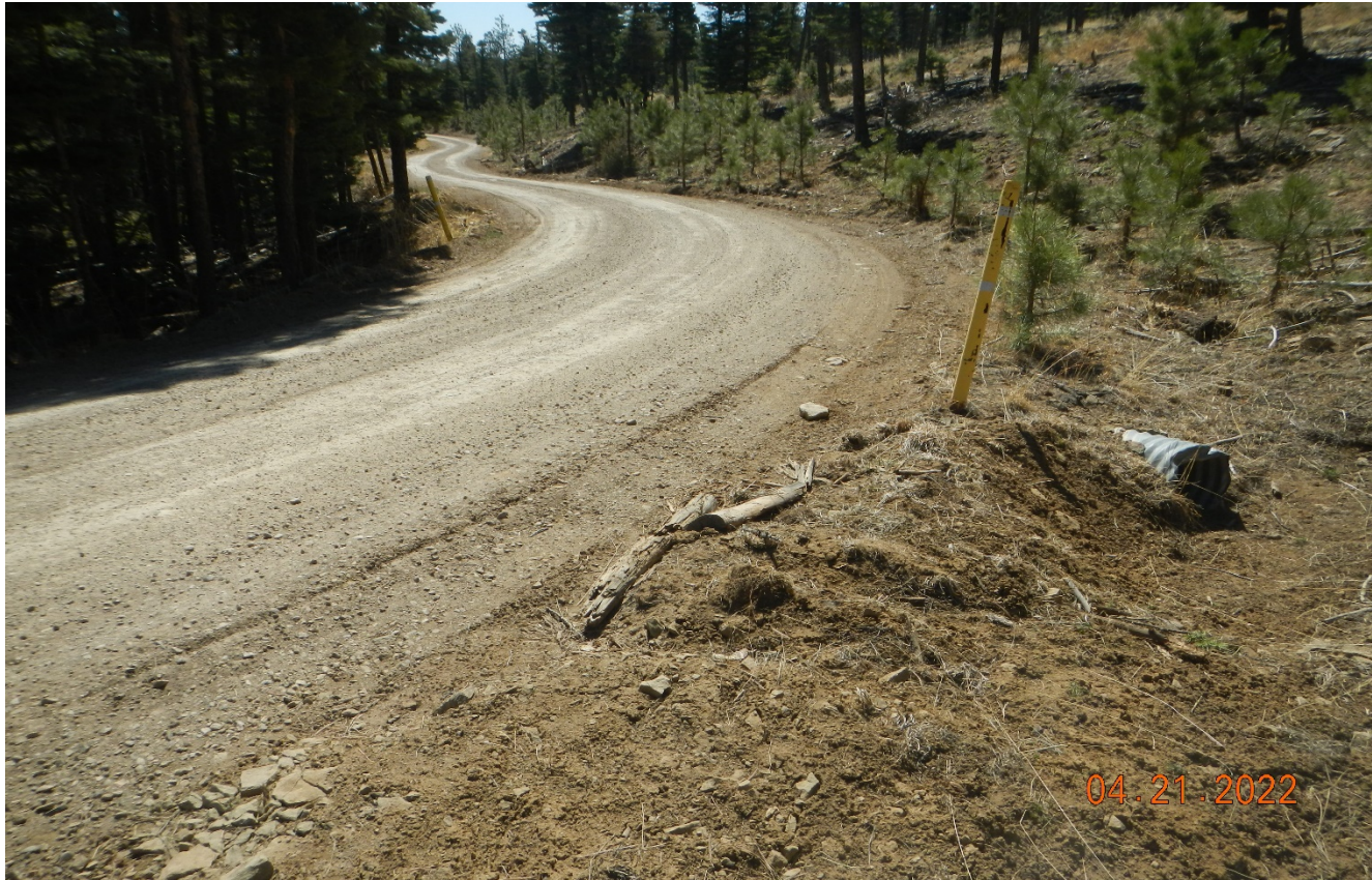
Photo 2. The culverts along the road have been cleaned out and maintained.
