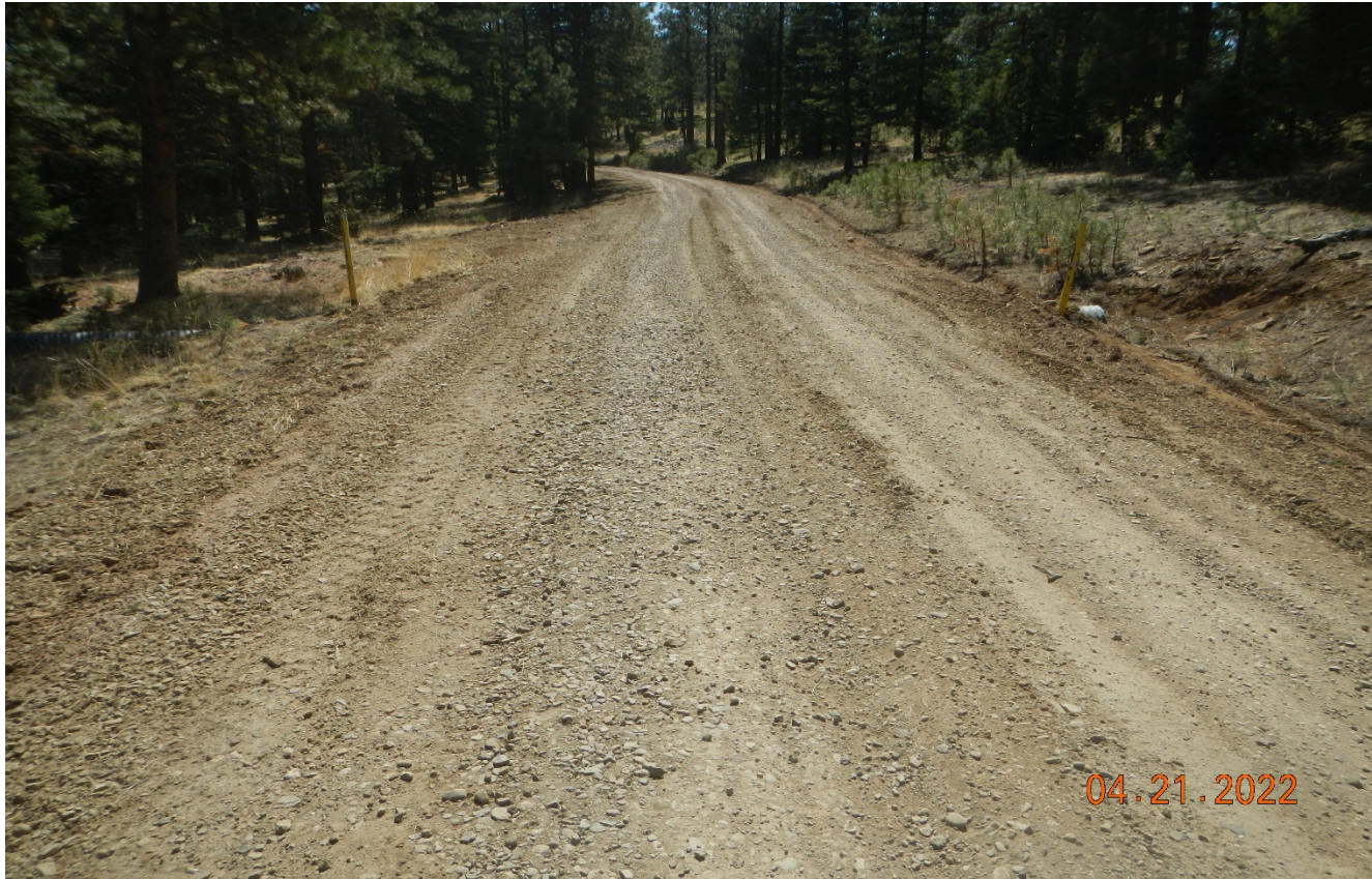
Photo 5. Facing southeast along the main access road. Additional gravel road base has been applied to areas of the road.
