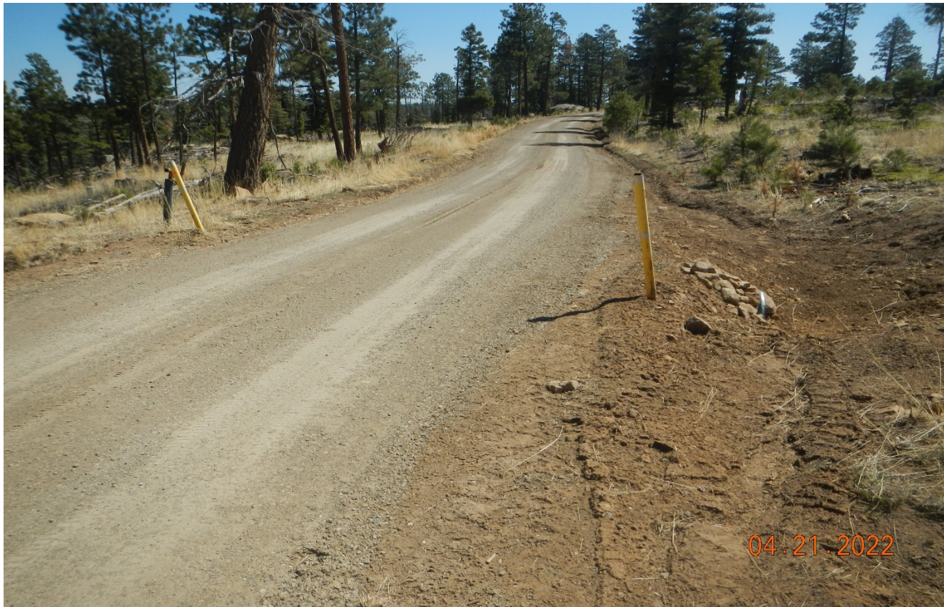
Photo 4. The culverts along the road have been cleaned out and maintained.
