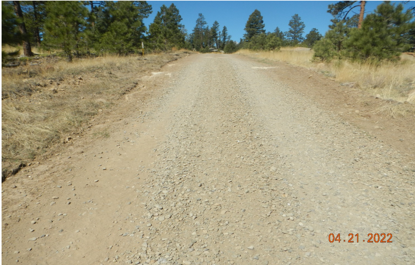
Photo 1. Facing west along the main access road. Additional gravel road base has been applied to areas of the road.
