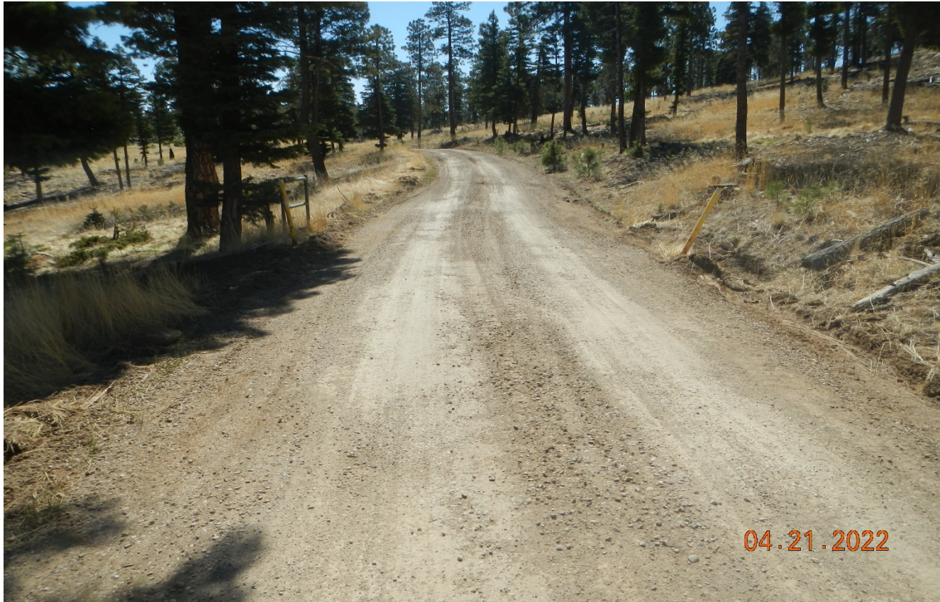
Photo 3. Facing southeast along the main access road. Additional gravel road base has been applied to low areas of the road where water would accumulate.
