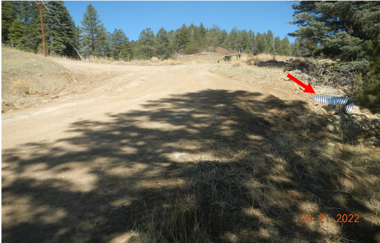
Photo 4. There was a new culvert installed near the location where frequent stormwater issues was observed.
