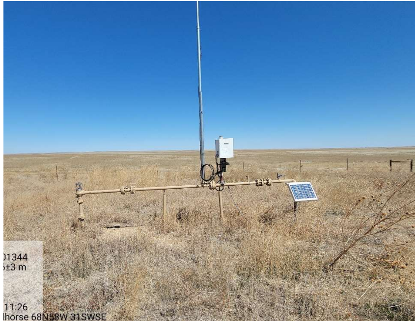
Photo 7 – Photo taken from the associated offsite tank battery, facing North. Photo illustrates the Operator has failed to perform final reclamation activities to remove all equipment.
