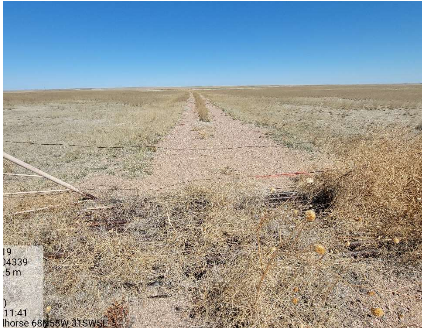
Photo 1 – Photo taken from the entrance of the well location, facing North. Photo illustrates the Operator has failed to perform final reclamation activities.
