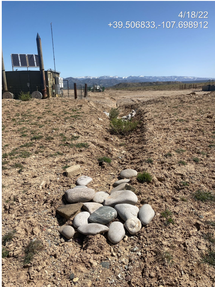
Photo 8. Photo taken from the south of the Location facing northeast shows a river rock lined sediment trap outlet.
