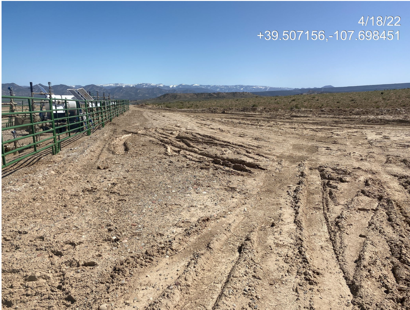
Photo 12. Photo taken from the south of the working pad area facing north shows signs of lack of stabilization BMPs in some areas (rutting is present) .
