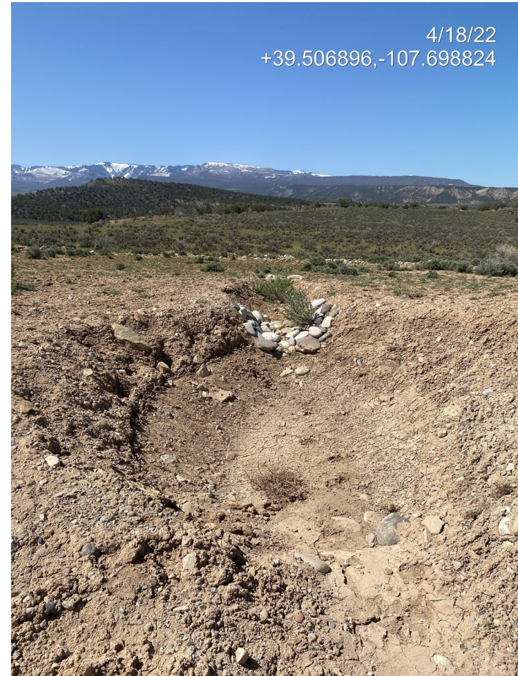
Photo 9. Photo taken from the south of the Location facing southwest shows a sediment trap which leads into a river rock lined outlet.
