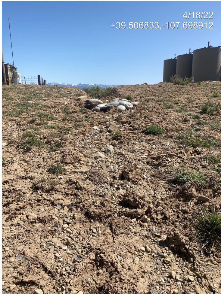
Photo 10. Photo taken from the south of the Location facing northeast shows pedestal formations due to stormwater degradation at a sediment trap outlet.
