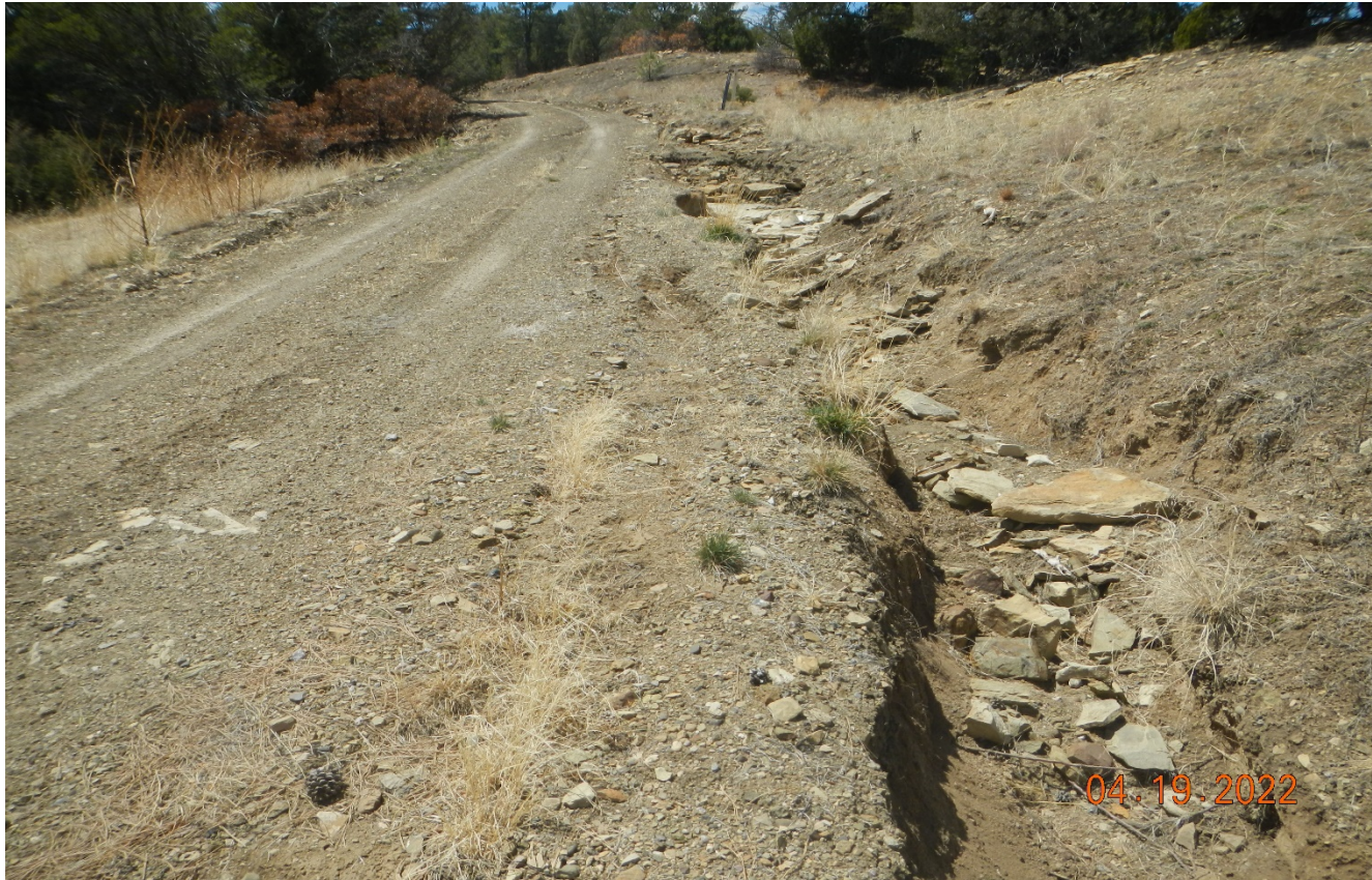
Photo 4. Facing southwest toward the access road. This area of erosion has not been repaired and stabilized. Previous corrective action was not completed.
