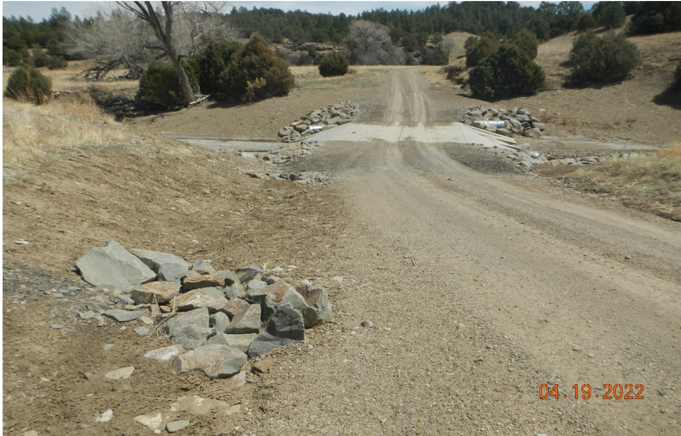
Photo 2. Facing east toward the access road stream crossing. The road side area was repaired and rock check dams were installed.
