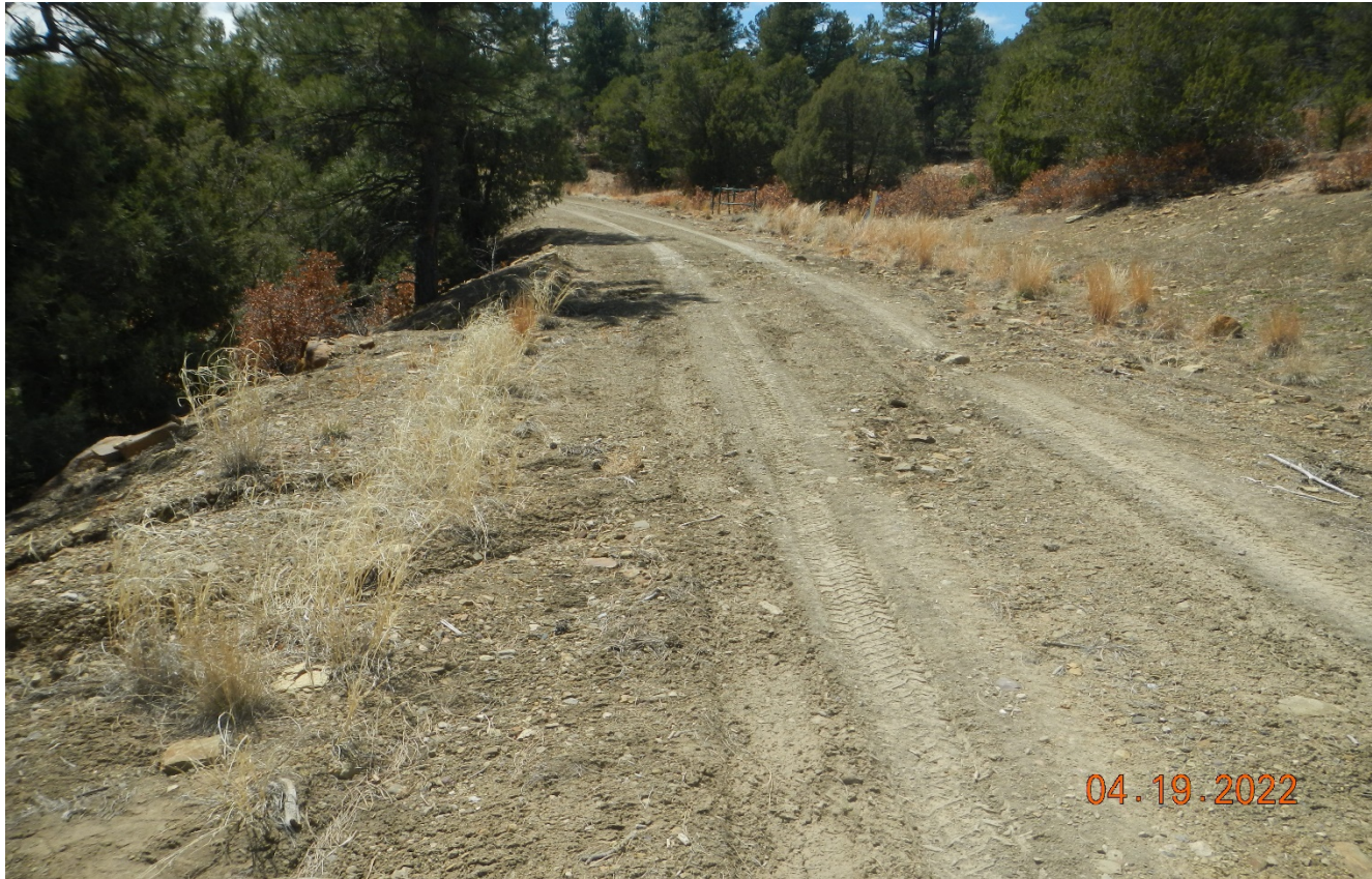
Photo 5. Further up the access road. There is stormwater erosion across the road. This area needs a culvert to prevent stormwater from eroding across the road and also further down the road side shown in previous photo.
