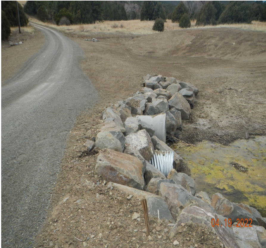
Photo 2. There are two culverts installed at the stream crossing. This appears to be inadequate as the prior cement culvert shown in the photo on the right had 3 large culverts.
