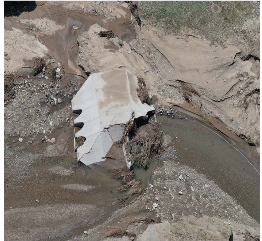
Photo 2. There are two culverts installed at the stream crossing. This appears to be inadequate as the prior cement culvert shown in the photo on the right had 3 large culverts.
