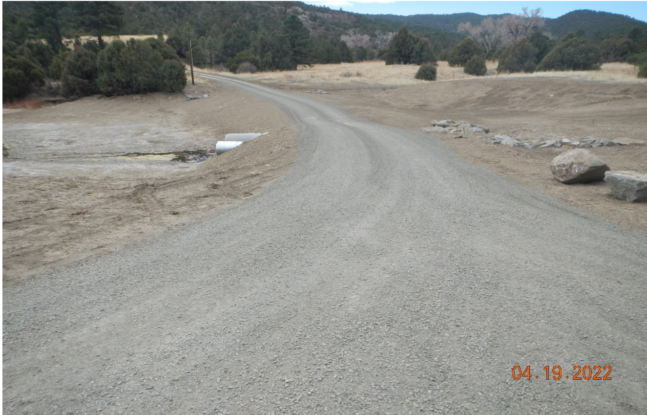
Photo 1. Facing south toward the access road stream crossing. There is no bank stabilization at the outlet side.
