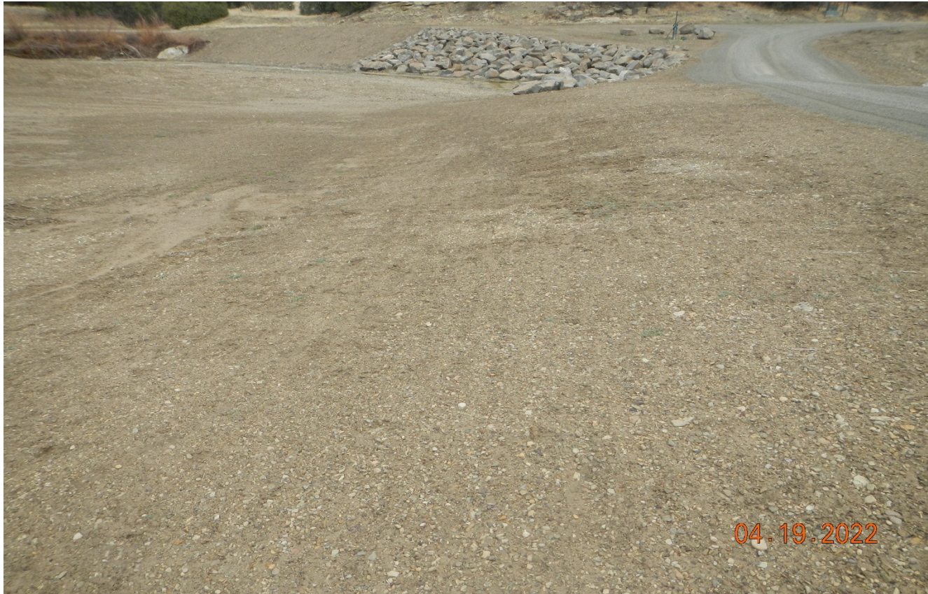
Photo 4. Facing northwest along the side of the access road. All disturbed areas along the road side need to be seeded and stabilized.
