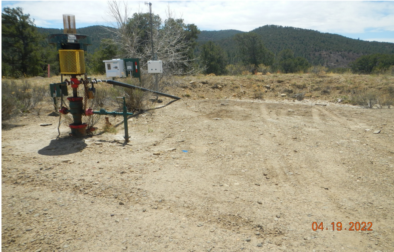
Photo 2. Facing toward the wellhead and pit.
