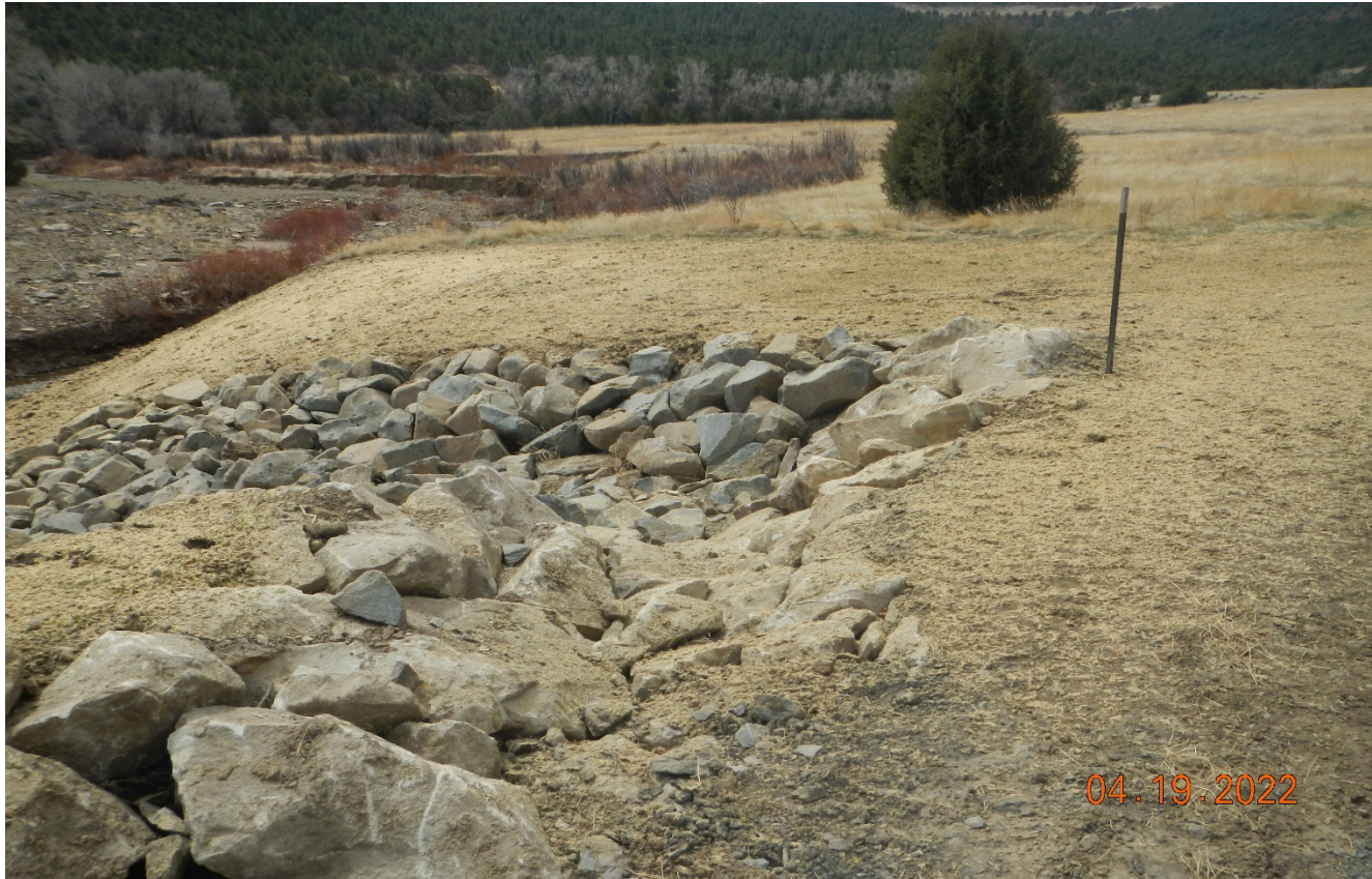
Photo 3. Further along the road the culvert outlet was repaired and rock outlet protection was installed.
