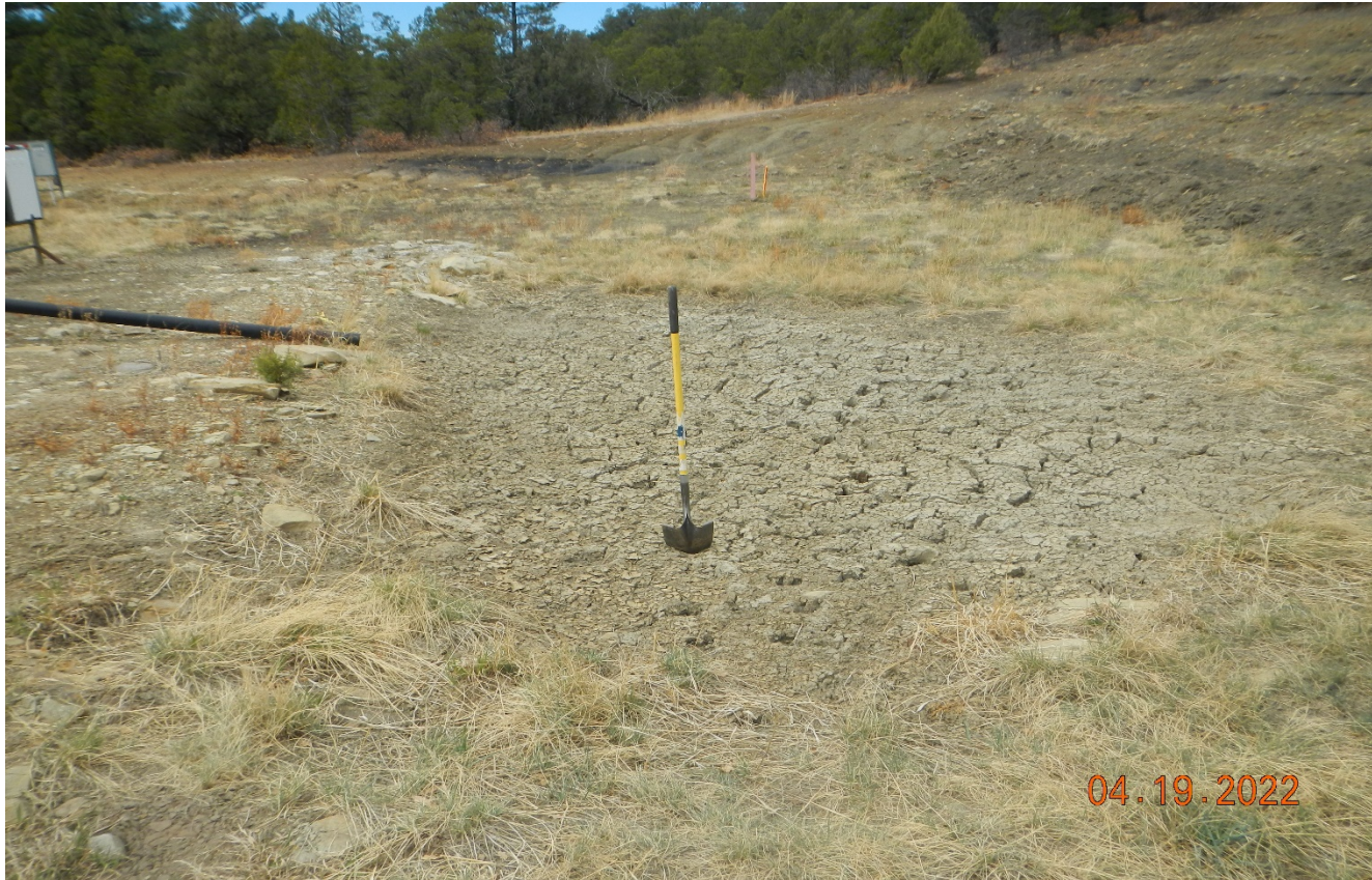
Photo 7. Facing toward the pit. Water level has been lowered. The pit is shallow <2 ft. deep and needs to be constructed to allow 2 ft. freeboard. Previous corrective action was not completed.
