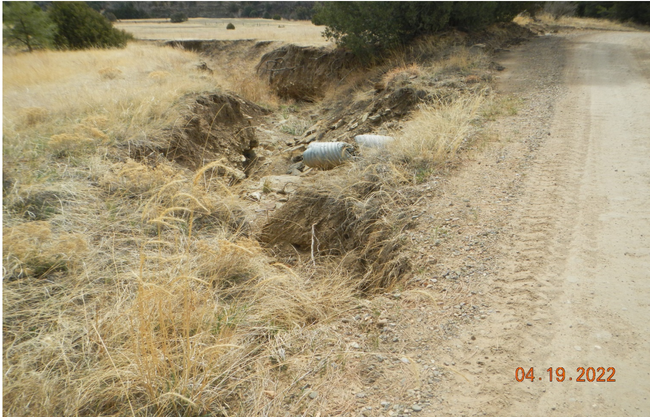
Photo 2. This culvert along the main road is partially washed out and needs to be repaired. Lat/Long:37.08136,-104.62910. This has not been repaired.
