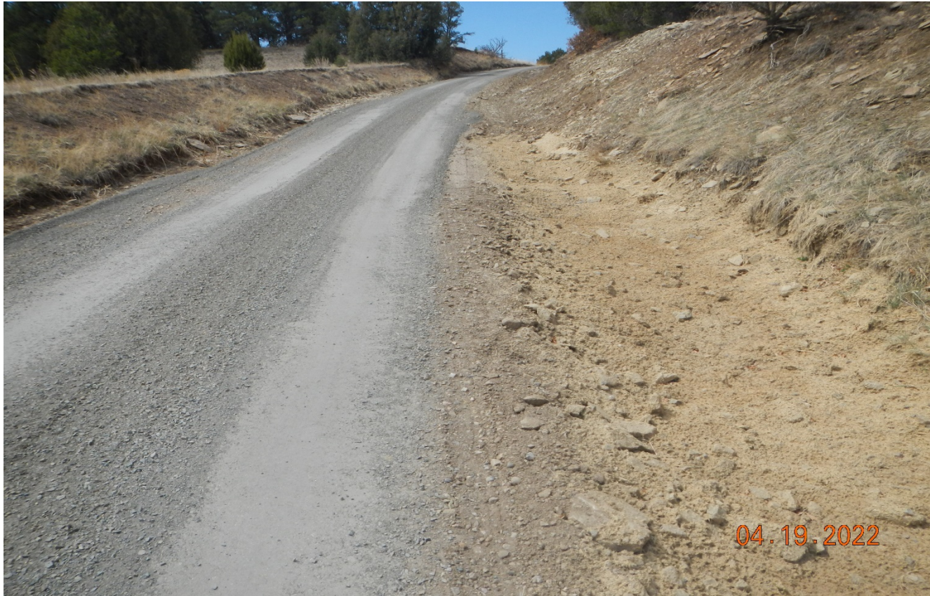
Photo 4. The road side has been repaired and stabilized.
