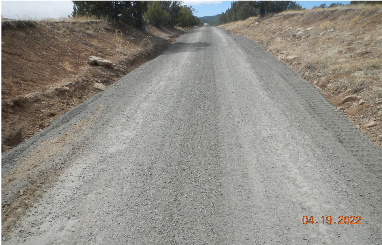
Photo 1. Facing southwest along the main road near the electric gate. There has been roadbase applied to this area of the road.
