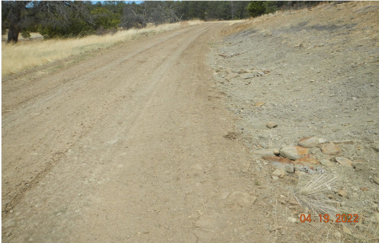
Photo 5. Further west along the access road. This area has been repaired. There are rock check dams installed however they are small and may not hold up very well.
