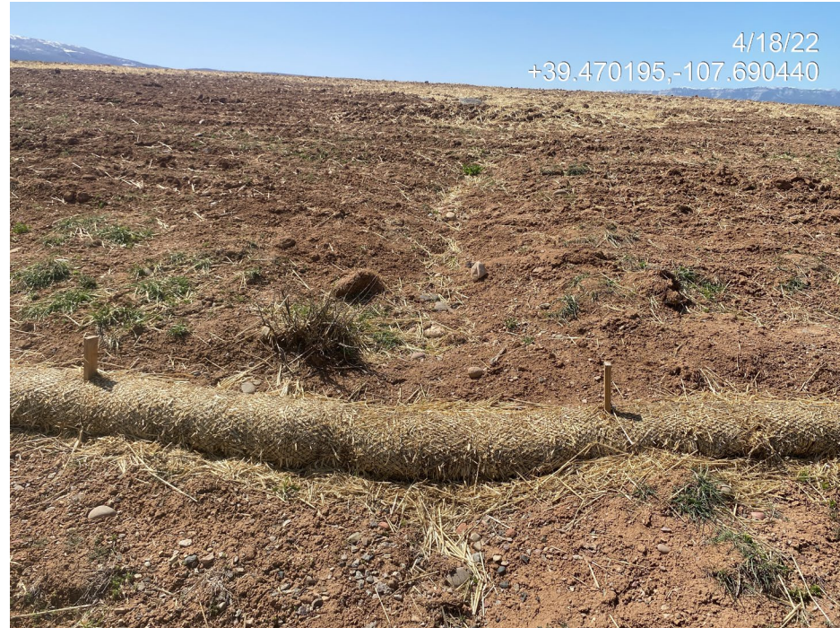
Photo 6. Photo taken from the northeast of the Location facing west shows a straw wattle on the perimeter of the Location.
