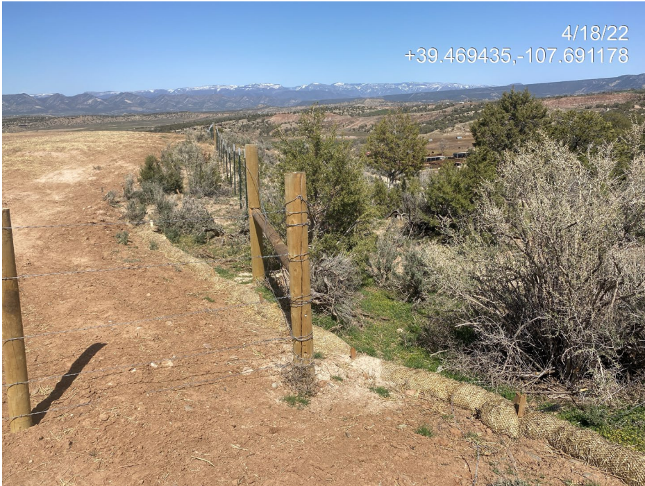
Photo 5. Photo taken from the southeast of the Location facing north shows a straw wattle on the perimeter of the Location.
