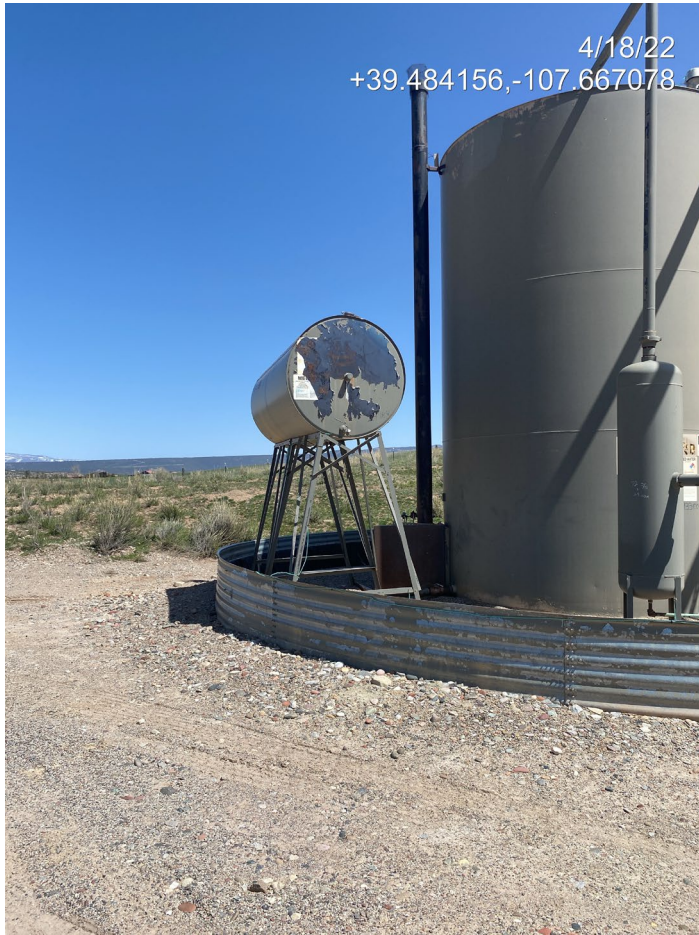
Photo 2. Photo taken from the tank battery shows the label on a methanol tank in disrepair.
